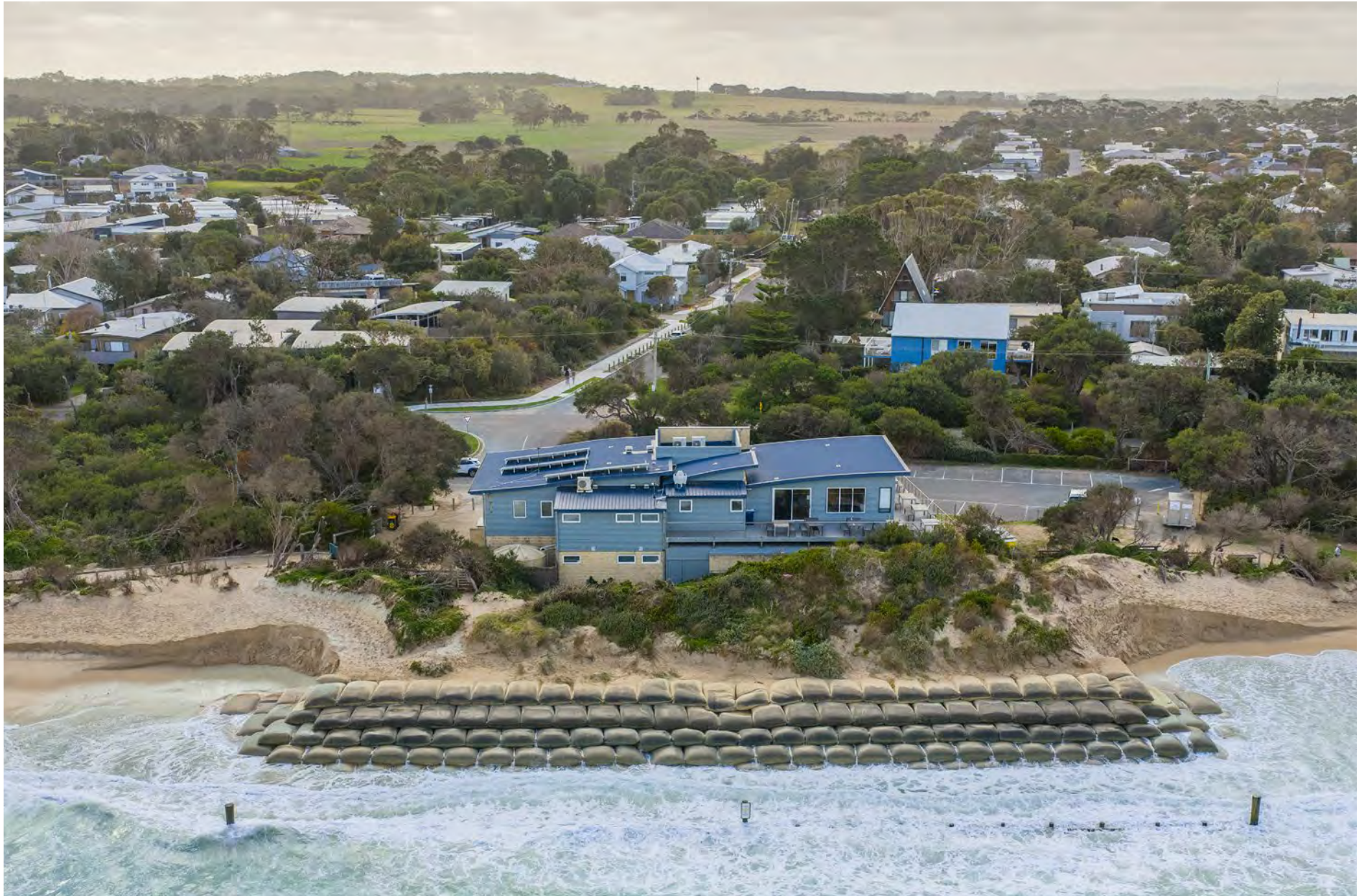
Image 9: This surf lifesaving club in Inverloch in Victoria's south-east is under threat from coastal erosion.
