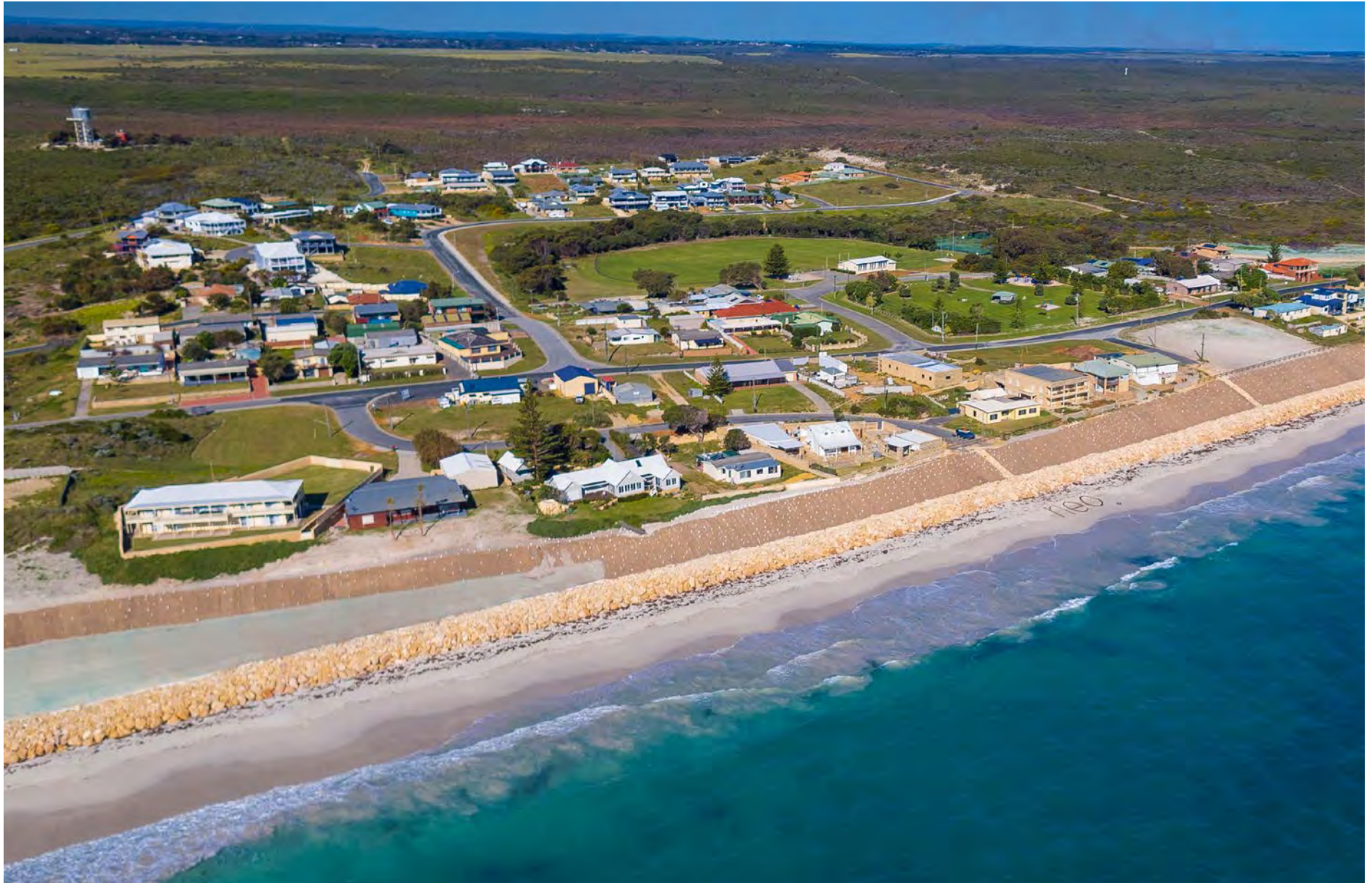
Image 7: This seawall of nearly 600 metres is currently protecting 15 homes and a public reserve from coastal flooding in Seabird, WA. However, with only a 20 year lifespan, this is far from a permanent solution to sea level rise for this community.
