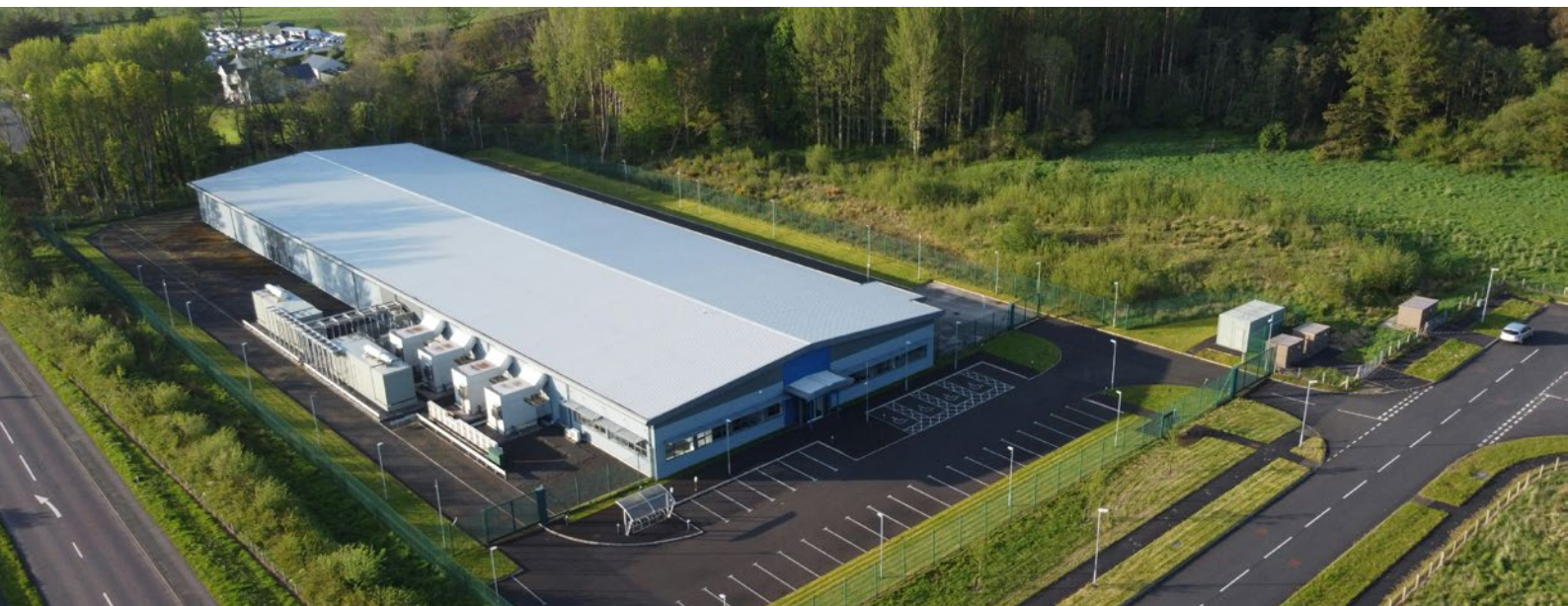
Image 2: Several major AI and cloud companies have recently announced significant Australian investments or expansions: Data centre in Coleraine, Victoria.
