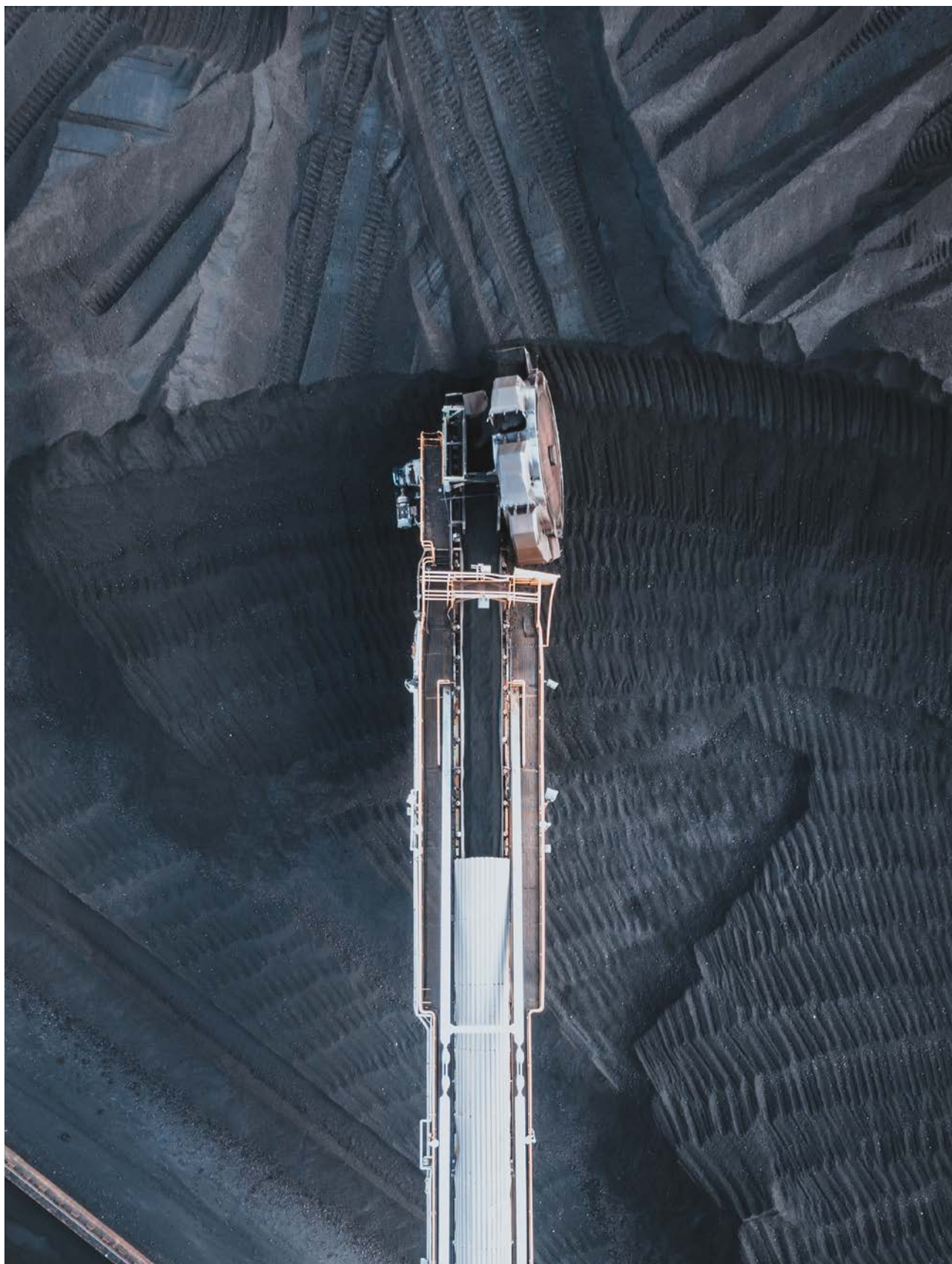
Figure 11: Coal moving on conveyor belts.
