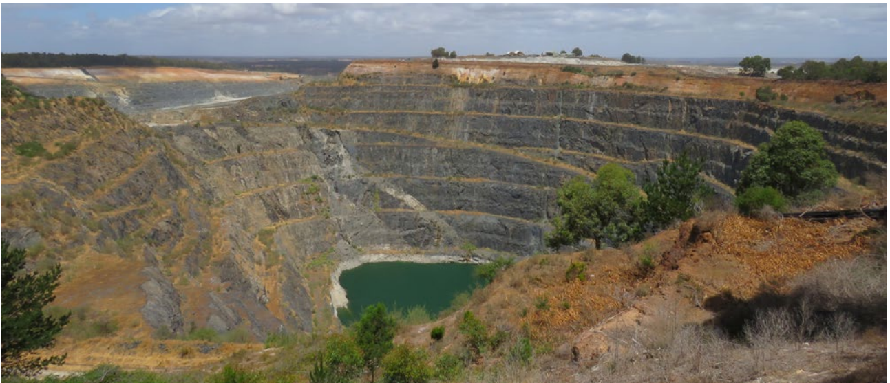
Figure 11: The Greenbushes lithium mine in the town of Greenbushes, Western Australia. Operational for over 30 years, the mine is undergoing the construction of a third lithium processing plant and retreatment facility (Talison Lithium, 2021).
