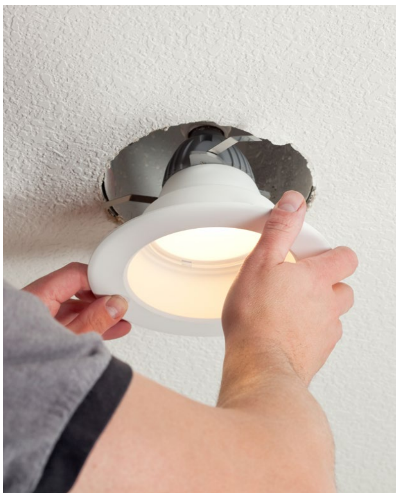
Image 1. Smarter lighting: Installing LED globes or replacing halogen downlights with LEDs can save up to 80 percent of lighting electricity costs.
