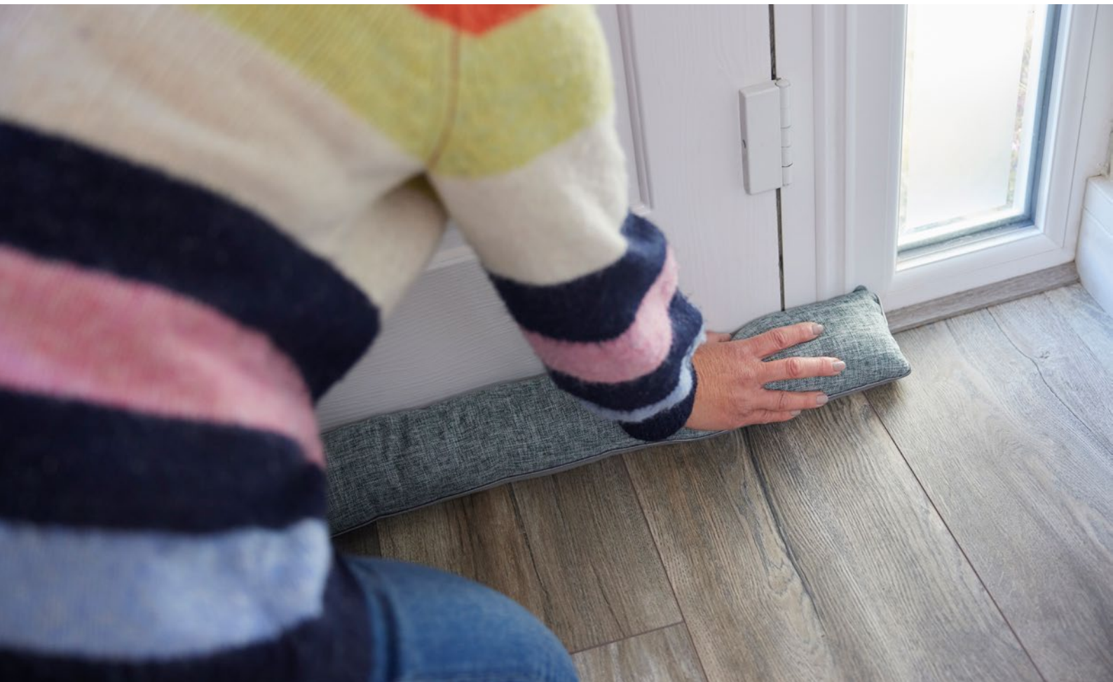
Image 5. Low-cost options: Draught sealing can be as simple as blocking gaps under doors using low-cost products that are widely available and moveable.
