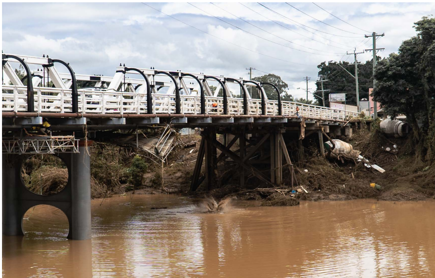
Figure 14: Road bridge badly damaged in Lismore in early 2022. The Feb-March floods in New South Wales badly damaged transport infrastructure costing at least $1.5 billion.
