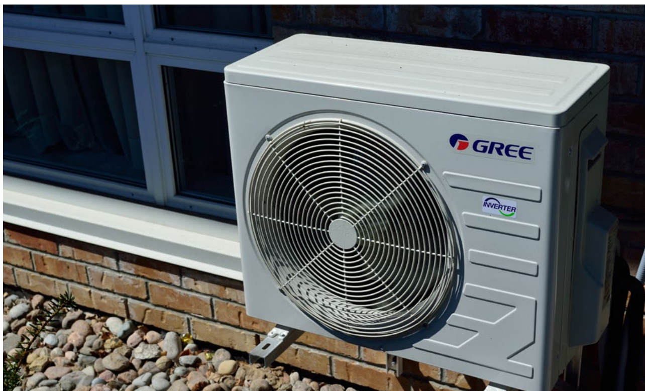
Figure 3: Air source heat pumps are the most common type of heat pump. The number installed in Australia has continued to increase over the years, from 7,822 in 2015 to 31,094 in 2020 (Statistica 2022).
