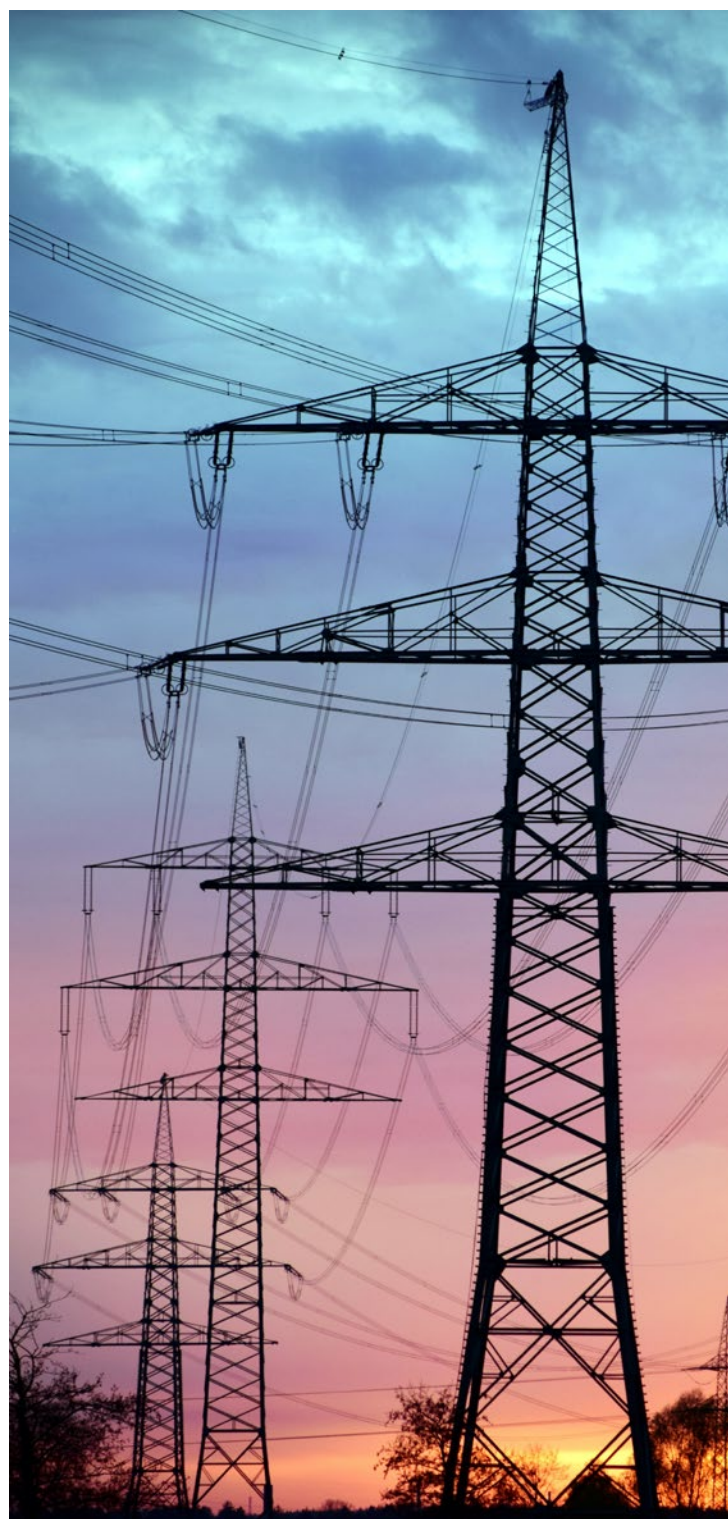
Figure 3: In February this year, construction began on Project EnergyConnect, a 900 kilometre transmission link between South Australia and New South Wales. It is the first of a number of key transmission lines proposed by the Australian Energy Market Operator to modernise the grid and support the rollout of renewables.
