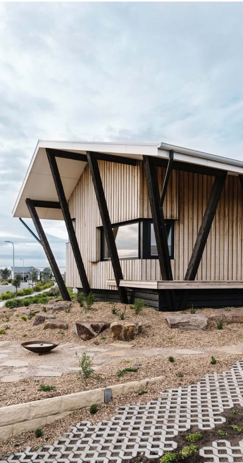
Figure 8: The Strait House in Cape Patterson, Victoria is built to an impressive 8.4 stars. Resident Richard Keech reflects “like anyone with lived experience of high-performing homes, we would find it very hard to go back to a home that doesn’t properly keep us comfortable. Everyone should expect more from their homes in this regard - it’s so much more than saving a few dollars on your energy bill.”
