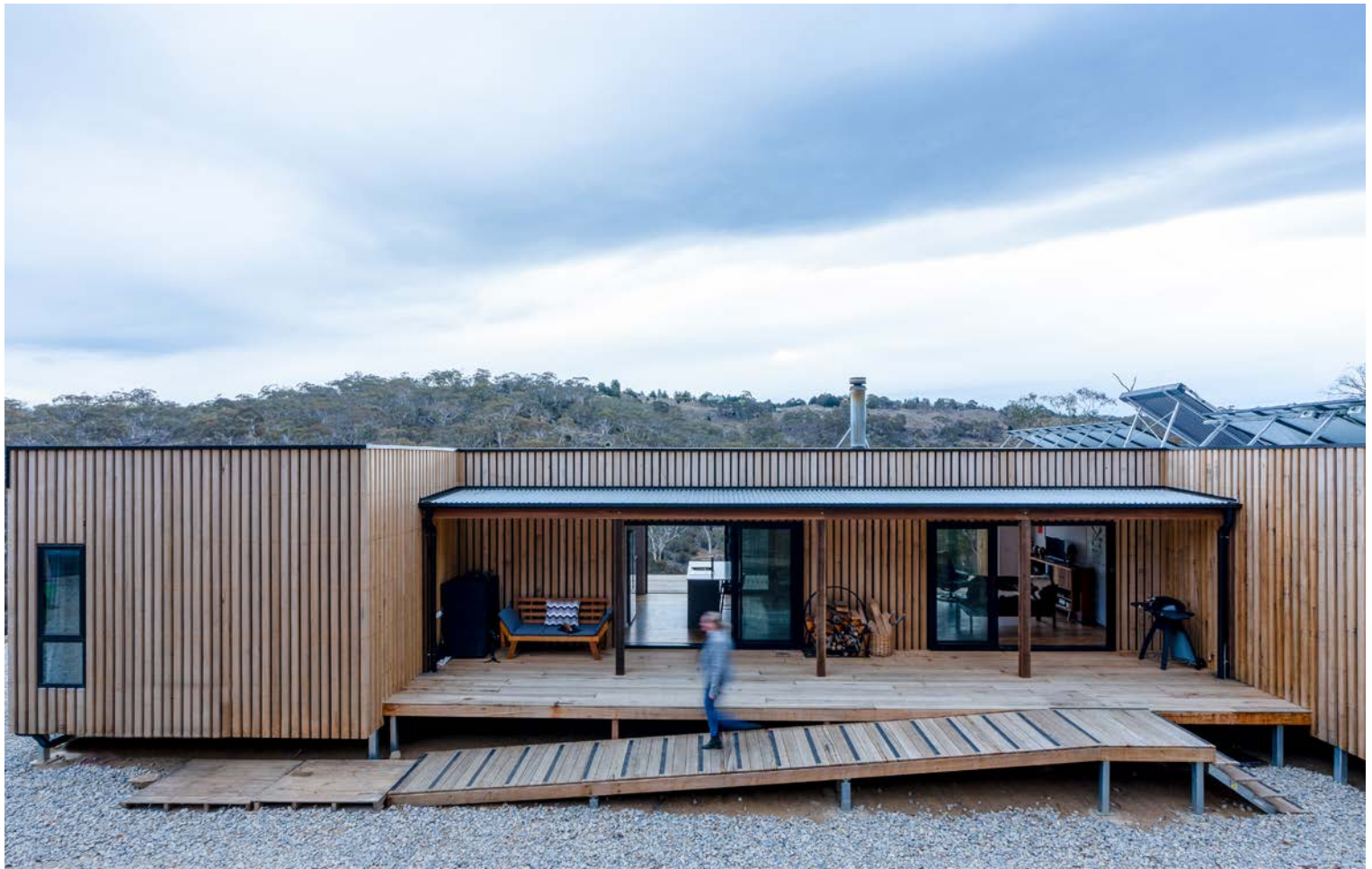
Figure 14: Even homes in remote locations can be built to higher energy efficiency standards. This 7-star home in Jindabyne, NSW is entirely off-grid and works to keep residents comfortable even in extreme summer and winter temperatures.
