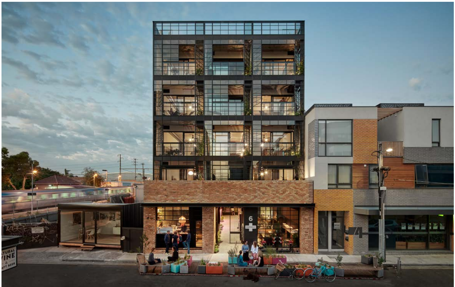
Figure 13: Ambitious developers are even seeking to exceed minimum standards in apartment buildings. Apartments in Nightingale 1 in Brunswick, Victoria achieve an average of 8.2-stars and operate on 100% renewable energy with no gas in the building.
