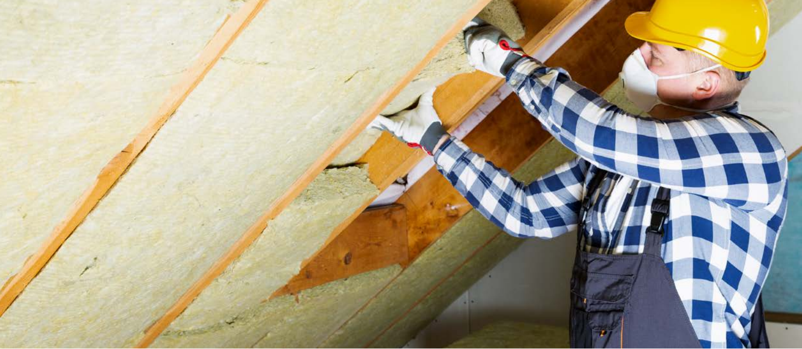
Figure 3: Insulation in ceilings, walls and underfloor can substantially reduce the energy (and cost) needed to heat and cool a house.
