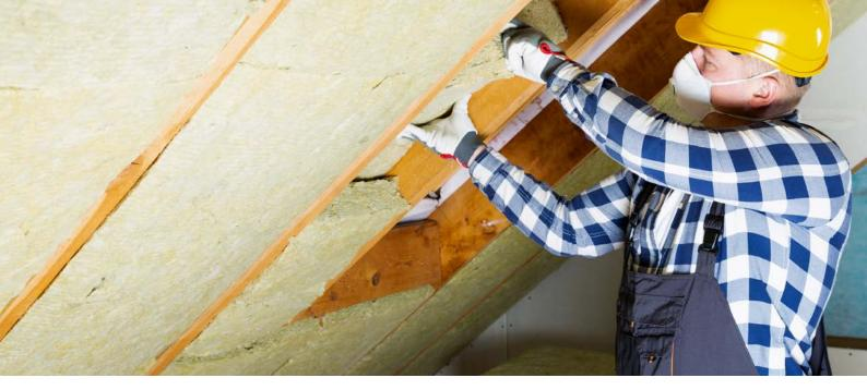
Figure 3: Insulation in ceilings, walls and underfloor can substantially reduce the energy (and cost) needed to heat and cool a house.
