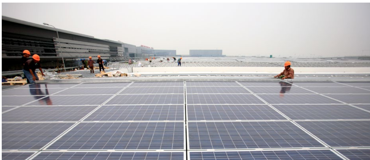
Figure 15: Installation of solar panels on the roof of the Hongqiao Passenger Rail Terminal in Shanghai, China.
