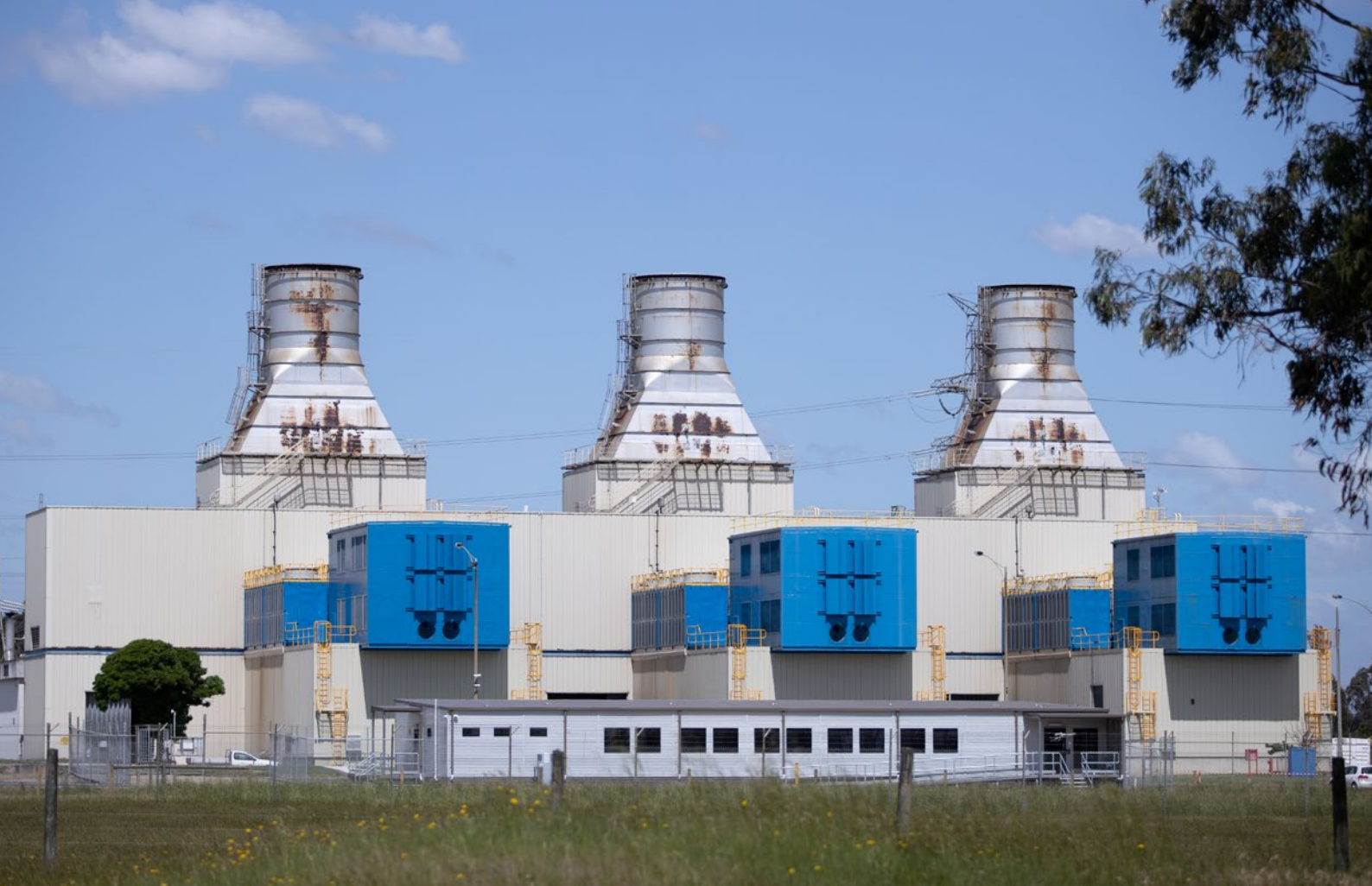
Figure 10: Australia's fleet of open-cycle generators, like Jeeralang B shown above, are very significantly less efficient than other forms of generation, and can be as emissions intensive as coal-fired generators.
