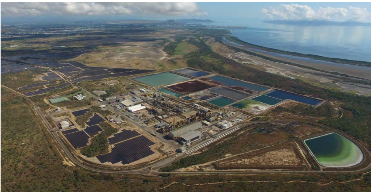
Figure 12: Sun Metals zinc refinery near Townsville installed a solar farm (pictured) to reduce costs and is now building a renewable hydrogen production facility onsite.
