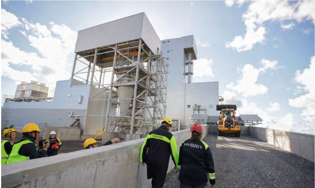
Figure 13: The HYBRIT project in Sweden is the world's first zero emissions steel pilot plant. Gladstone could be a key global player in clean steel manufacturing.
