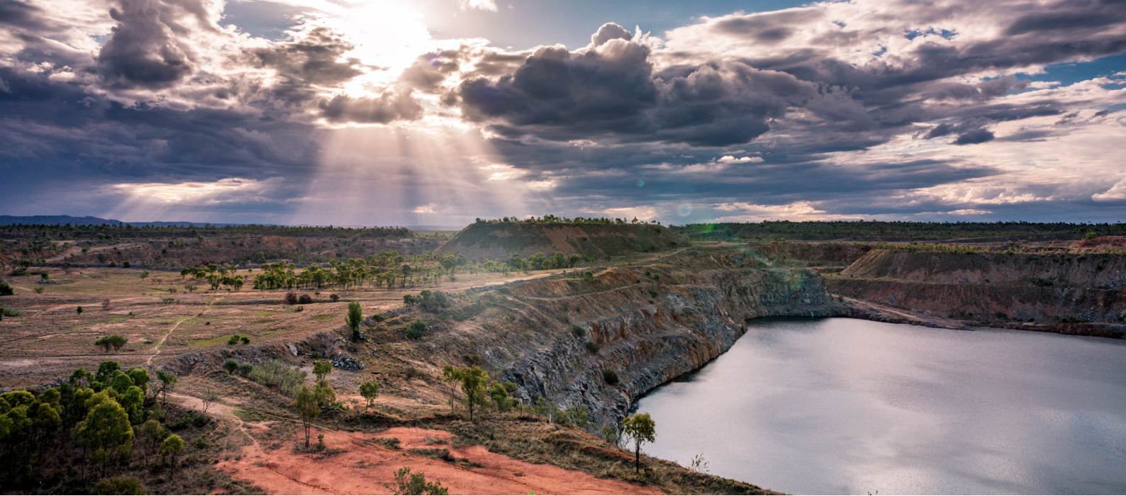
Figure 16: The 250MW Kidston pumped hydro project is converting an abandoned goldmine in north Queensland into a resource providing storage for renewables and dispatchable energy on demand.
