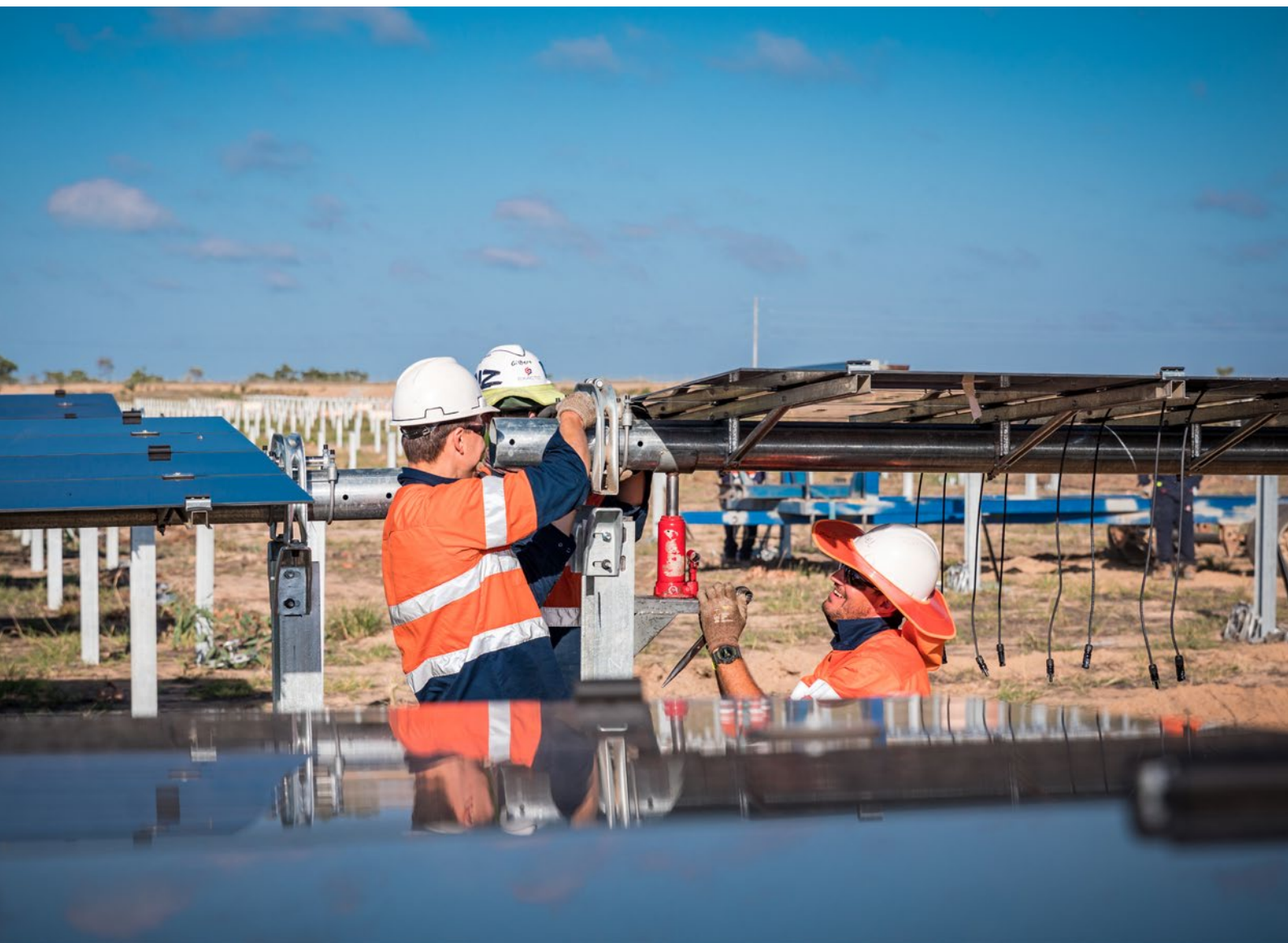
Figure 15: Workers installing solar panels on the Kidston solar farm, located north-west of Townsville in North Queensland. Renewable energy can create thousands of new jobs, especially in regional areas.
