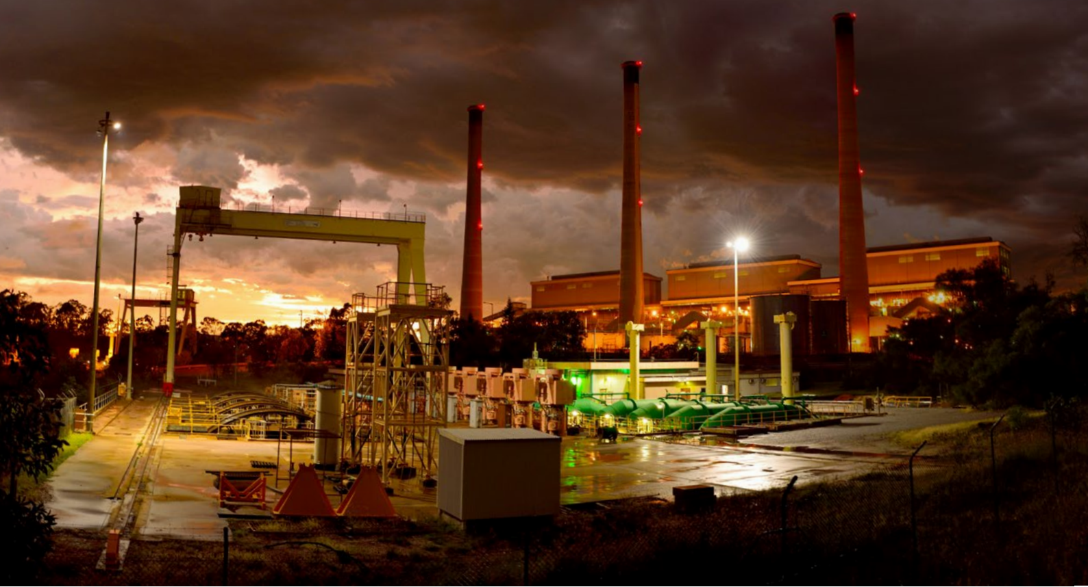
Figure 12: The Gladstone coal power station (pictured) released more oxides of nitrogen in 2017-18 than any other power station in Australia. Coal power stations have a range of negative human health impacts.
