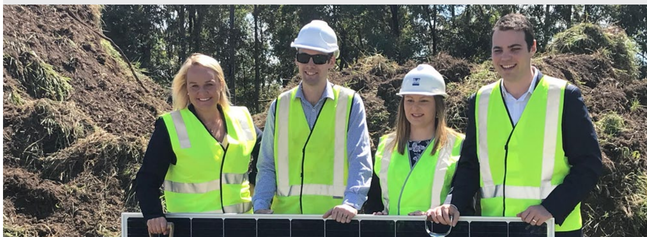
Figure 9: Construction on the Summerhill Waste Management Centre's solar farm began in November 2018 (pictured), supported by the City of Newcastle.
