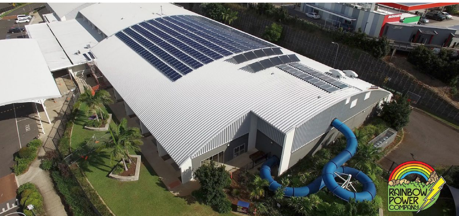
Figure 8: The Goonellabah community solar farm was supported by the Lismore City Council as part of its plan to be powered entirely by renewable energy by 2023.
