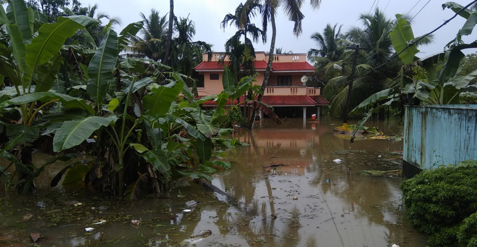
Figure 15: Kerala floods in India, August 2018.
