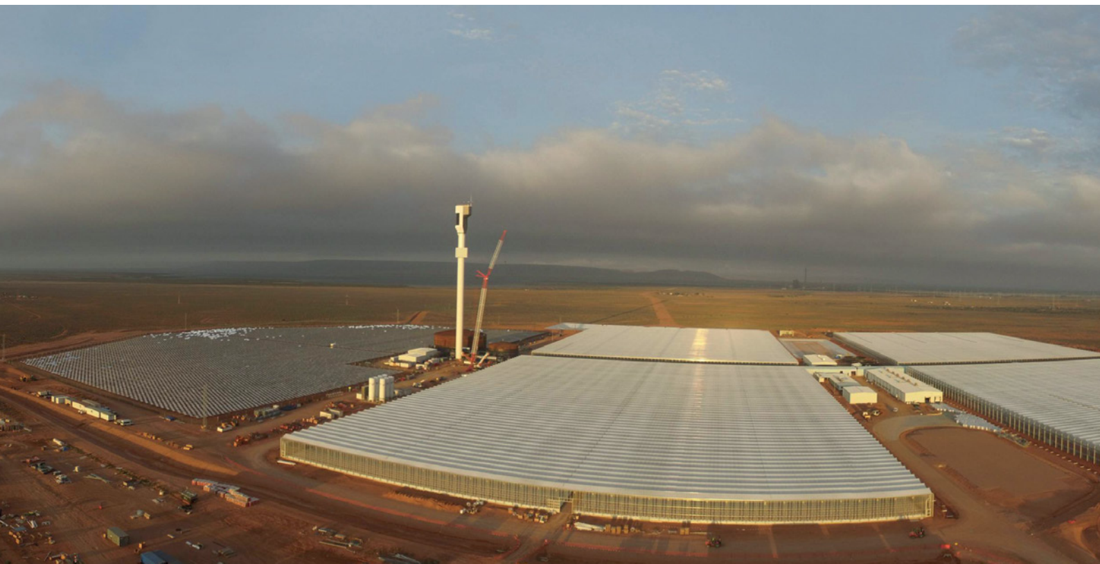
Figure 8: This solar thermal plant provides around 90% of the electricity needs of tomato growers Sundrop Farms in Port Augusta, South Australia.
