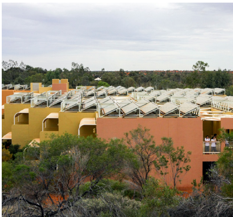
Figure 12: Solar panels on a hotel roof near Uluru, Northern Territory. 13.8% of households in the Territory have installed rooftop solar.
