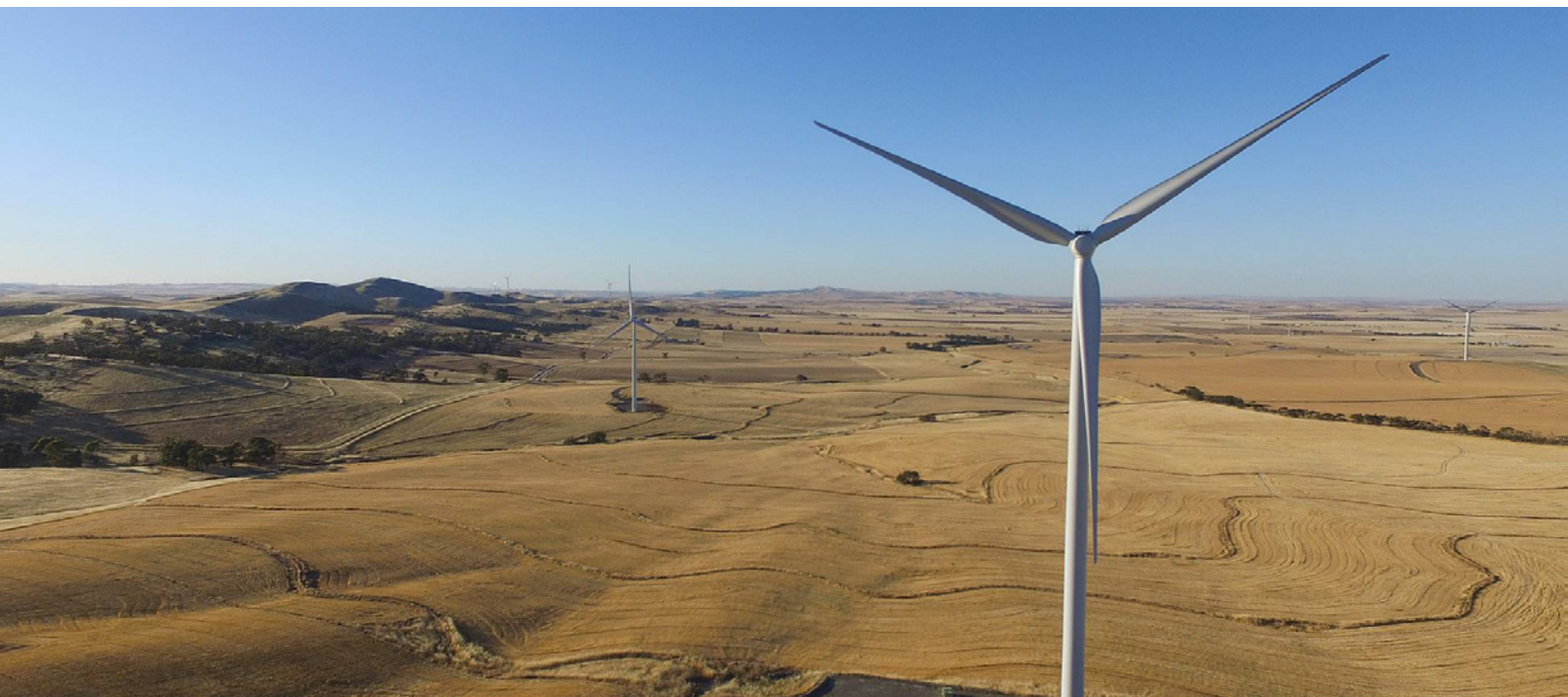
Figure 6: The three stages of the Hornsdale Wind Farm in South Australia (below) put forward winning bids under the ACT's reverse auction process. Stages 2 and 3 of the project set record low prices for wind energy in Australia at the time.
