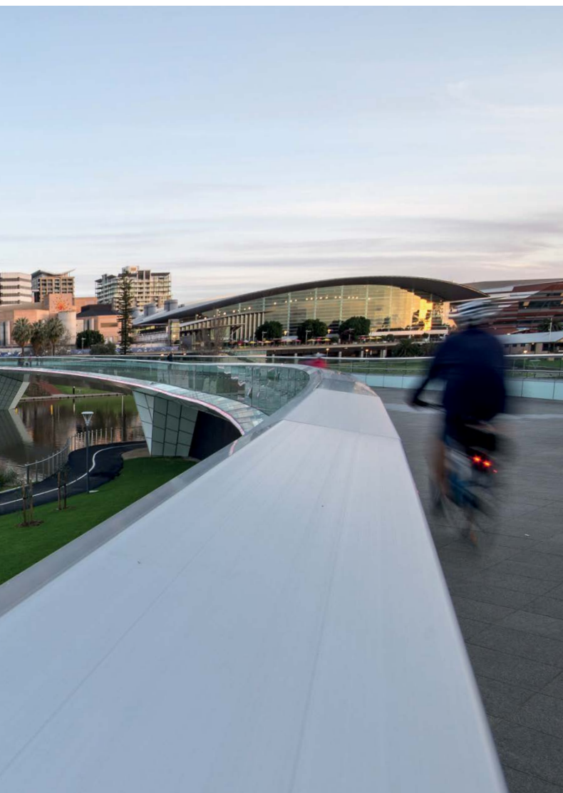
Figure 15: Adelaide Riverbank Pedestrian Bridge.
