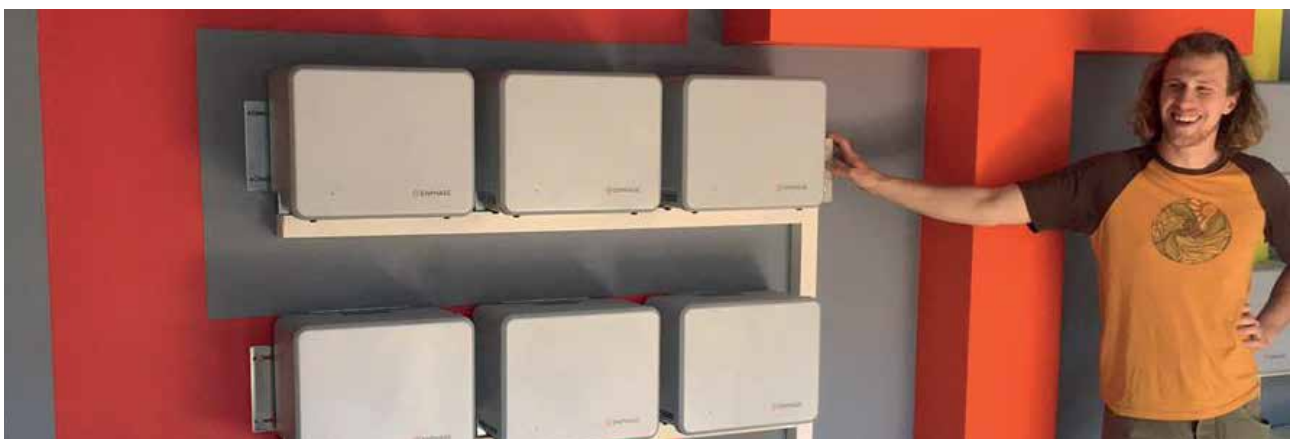
Figure 13: A battery storage installation in Sydney's Stucco apartments.
