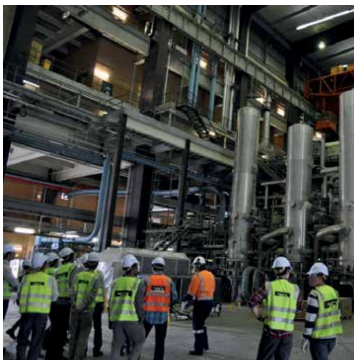
Figure 18: Inside South Australia’s Torrens Island gas power station.
