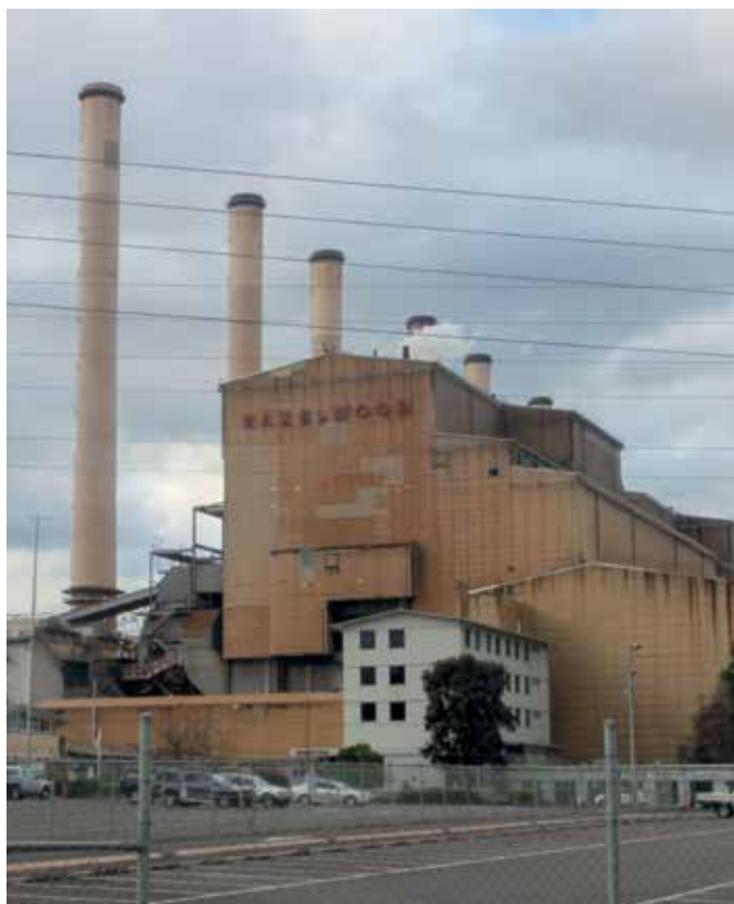
Figure 20: The Hazelwood coal power station, whose owners provided just six months notice before closing the power station in March 2017.
