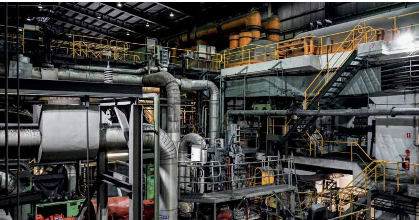
Figure 23: The interior of the ageing Liddell coal fired power station.
