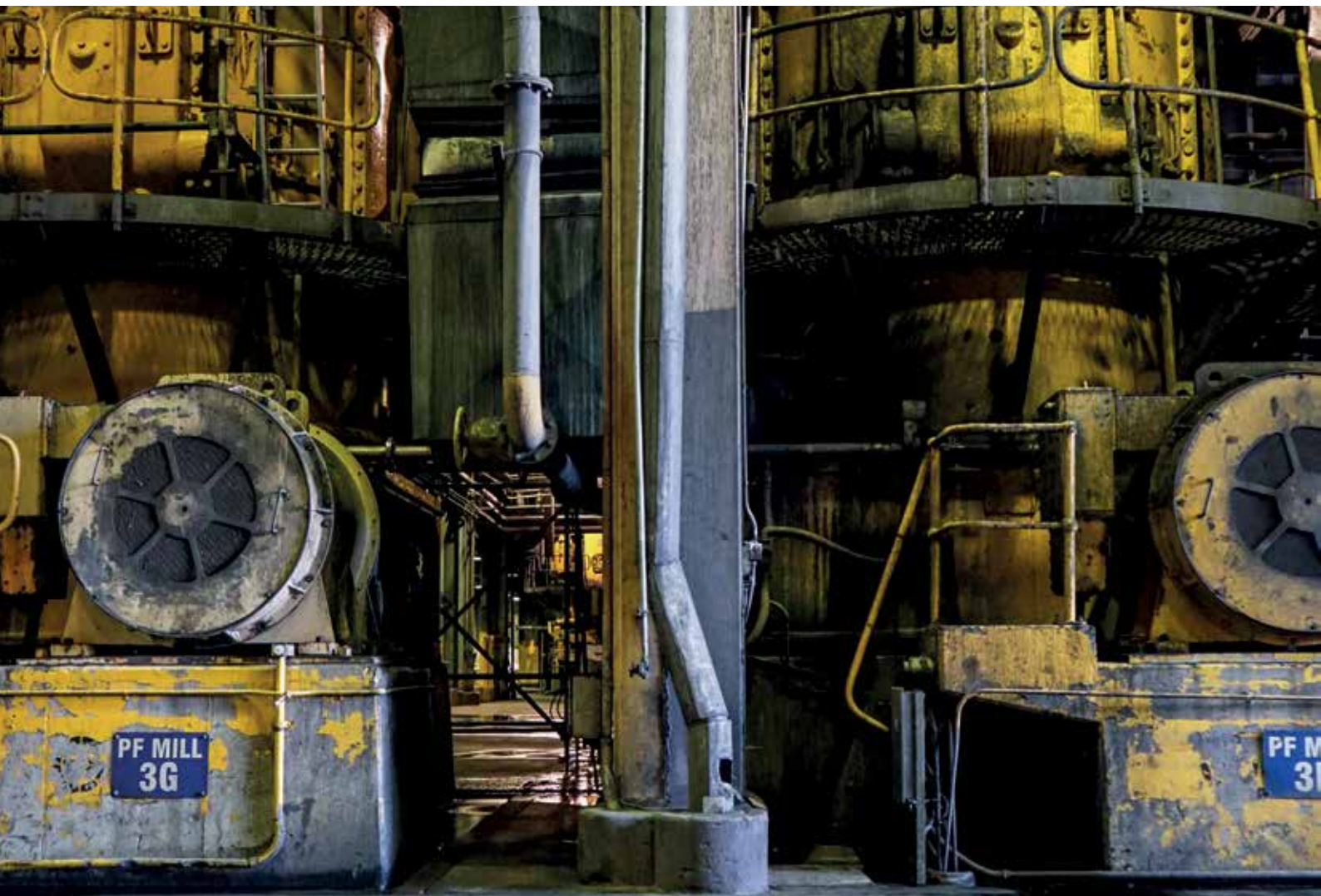
Figure 15: Inside New South Wales' ageing Liddell coal fired power station.
