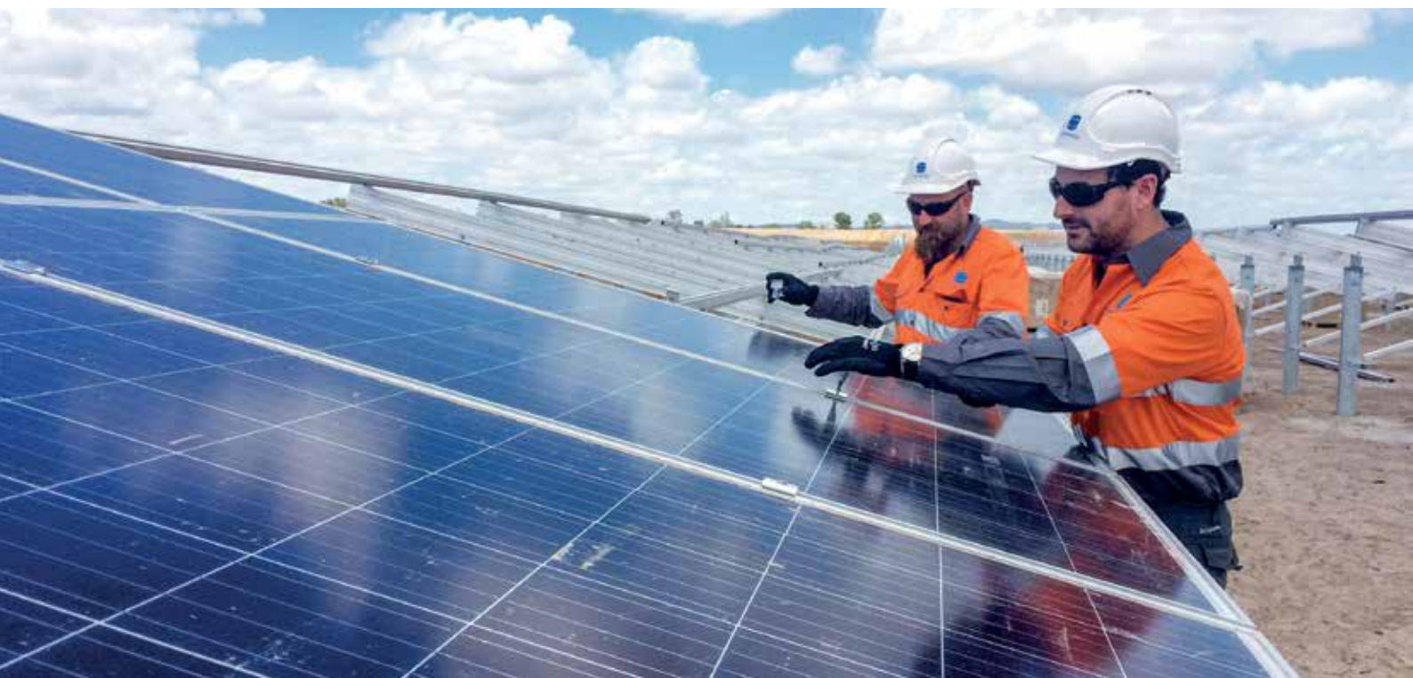
Figure 11: The Lakeland integrated solar and battery storage farm is the Southern Hemisphere's first large-scale integrated solar and battery storage facility.
