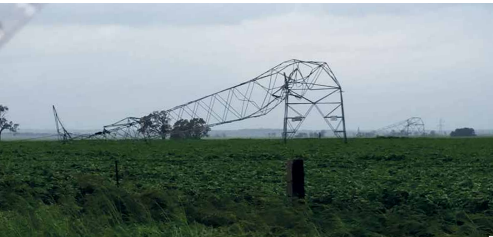
Figure 1: Severe storms in South Australia brought down transmission towers in 2016.
