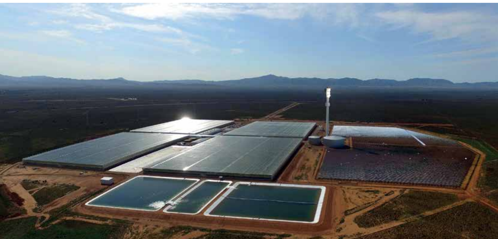
Figure 12: Sundrop Farms have built a solar thermal plant to power their tomato growing business in Port Augusta, South Australia.
