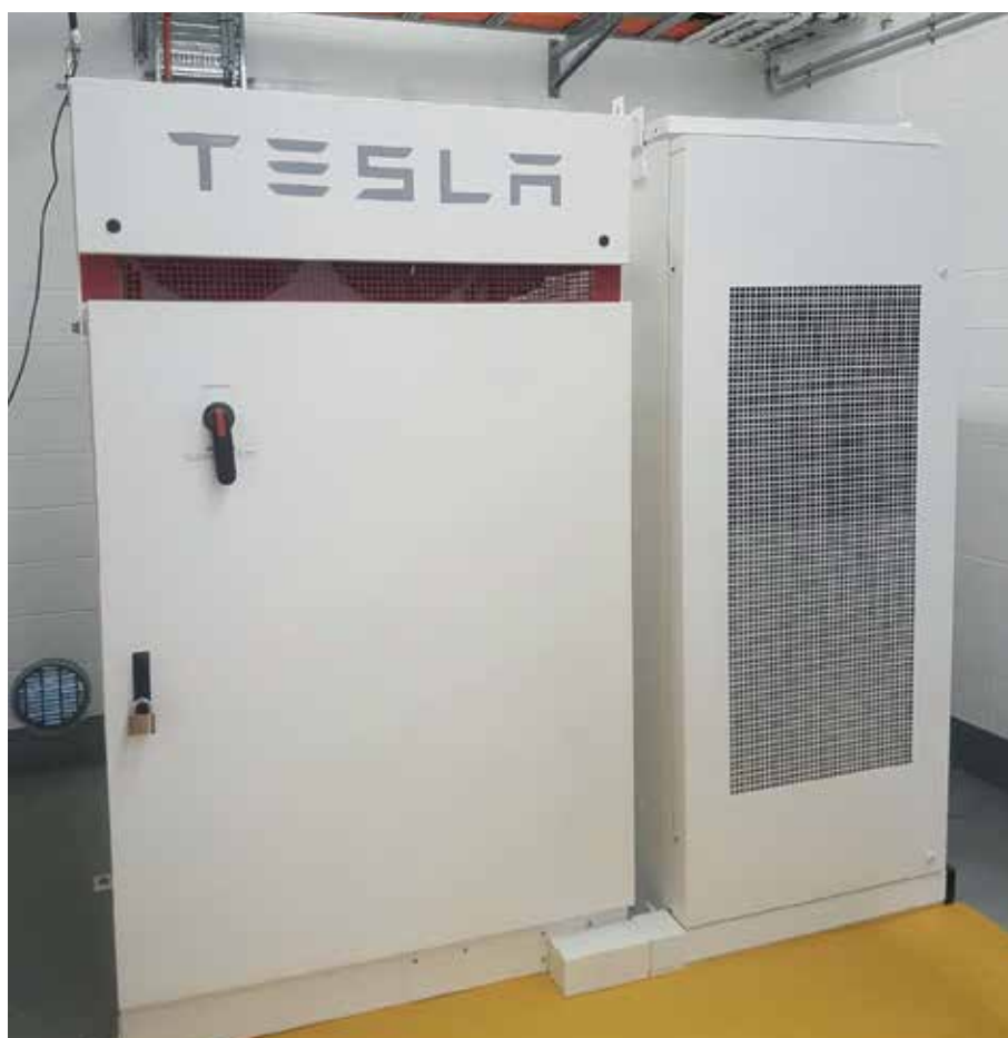
Figure 14: The Logan City Council battery storage system. Along with attached solar panels, the battery will reduce the council's energy costs by $50,000 per year.
