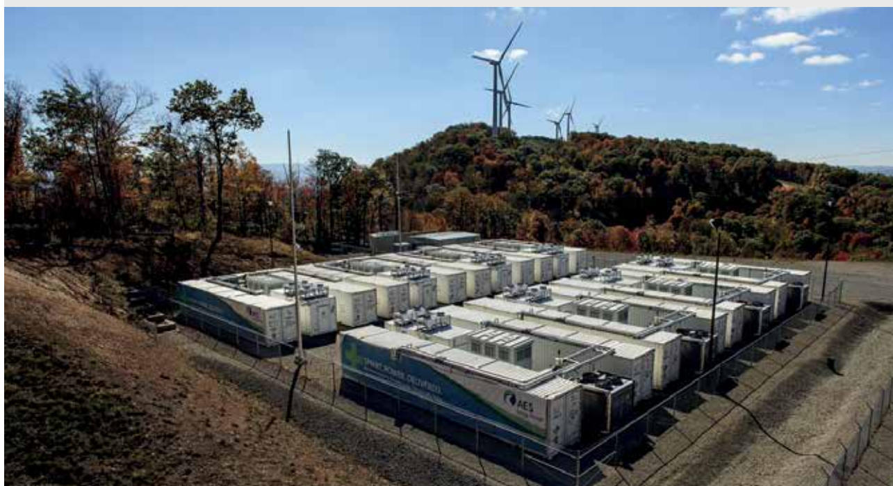
Figure 15: The 32MW Laurel Mountain battery farm in West Virginia, USA. The installation consists of lithium-ion batteries that store power from a nearby wind farm.
