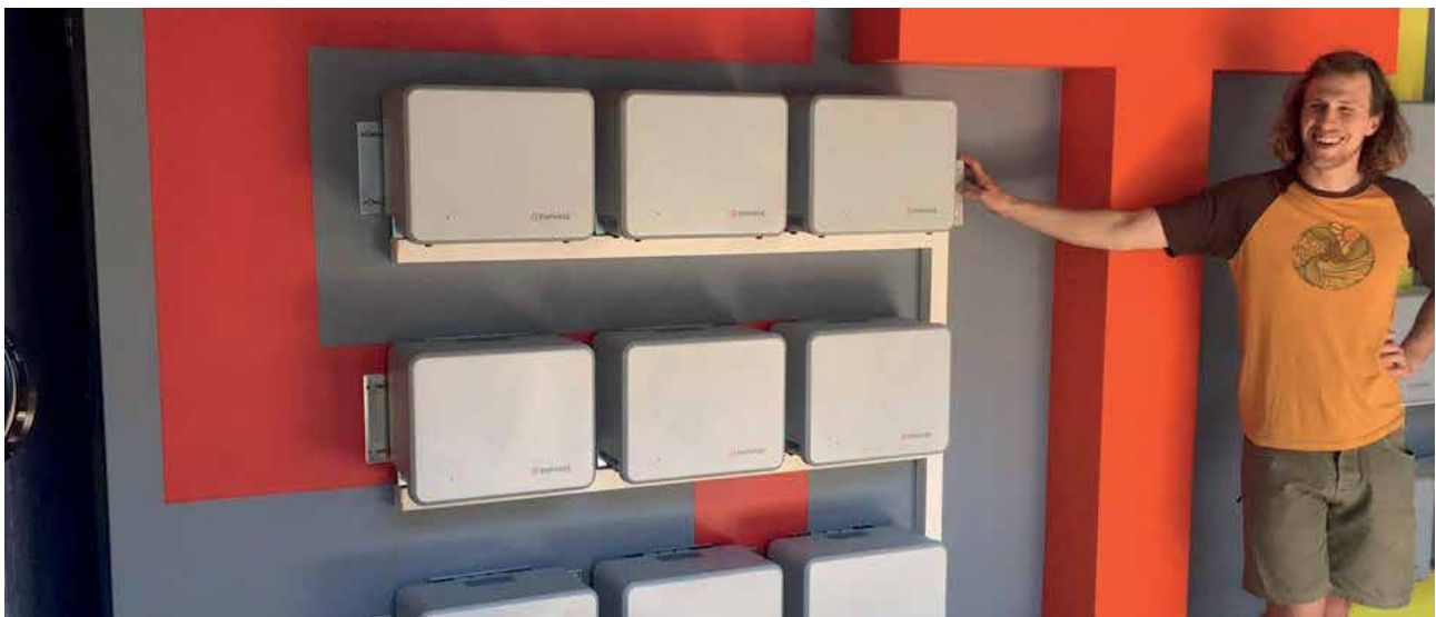
Figure 6: A battery storage installation in Sydney's Stucco apartments. Batteries are modular and can be upscaled or downscaled depending upon the quantity of storage that is required.
