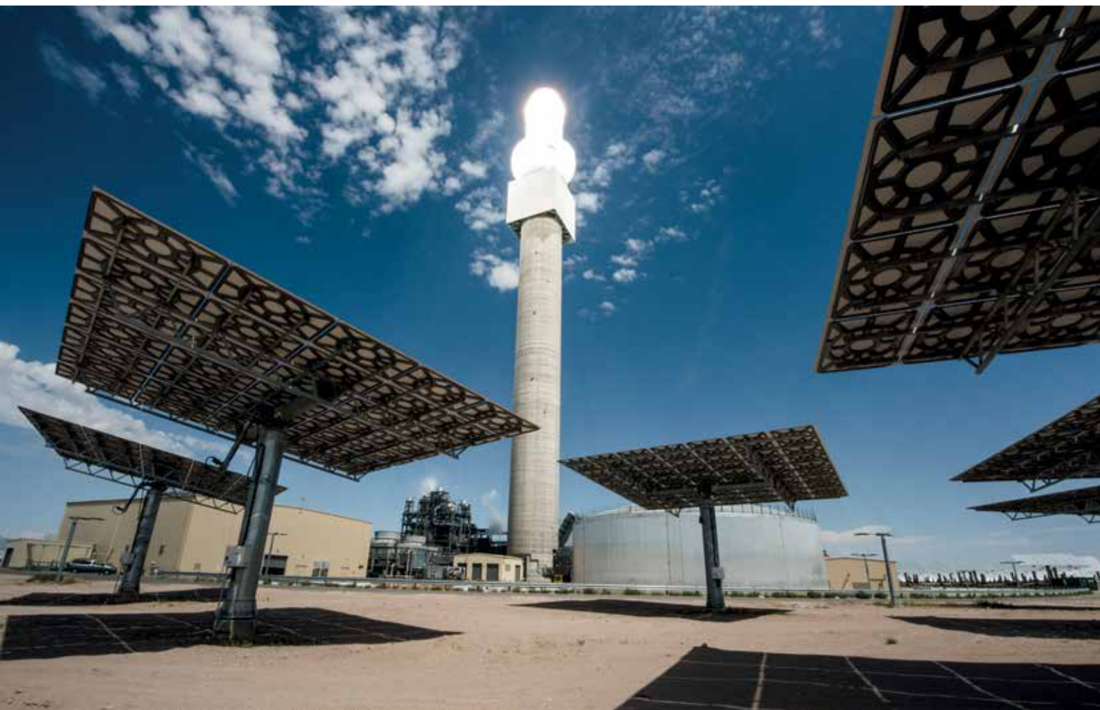
Figure 8: Crescent Dunes solar thermal farm in Nevada. Solar thermal farms store the energy they produce, so they can provide reliable power 24/7.
