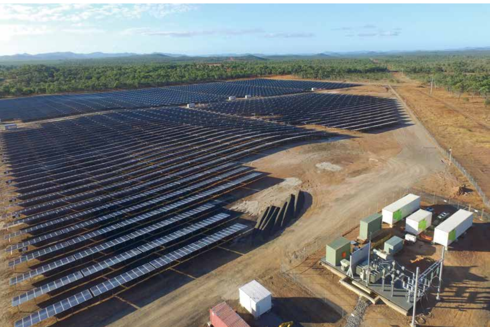
Figure 18: The Lakeland solar and storage facility. This is the Southern Hemisphere's first large-scale solar and battery storage installation. The batteries (bottom left) will enable the facility to provide a steady supply of reliable power.
