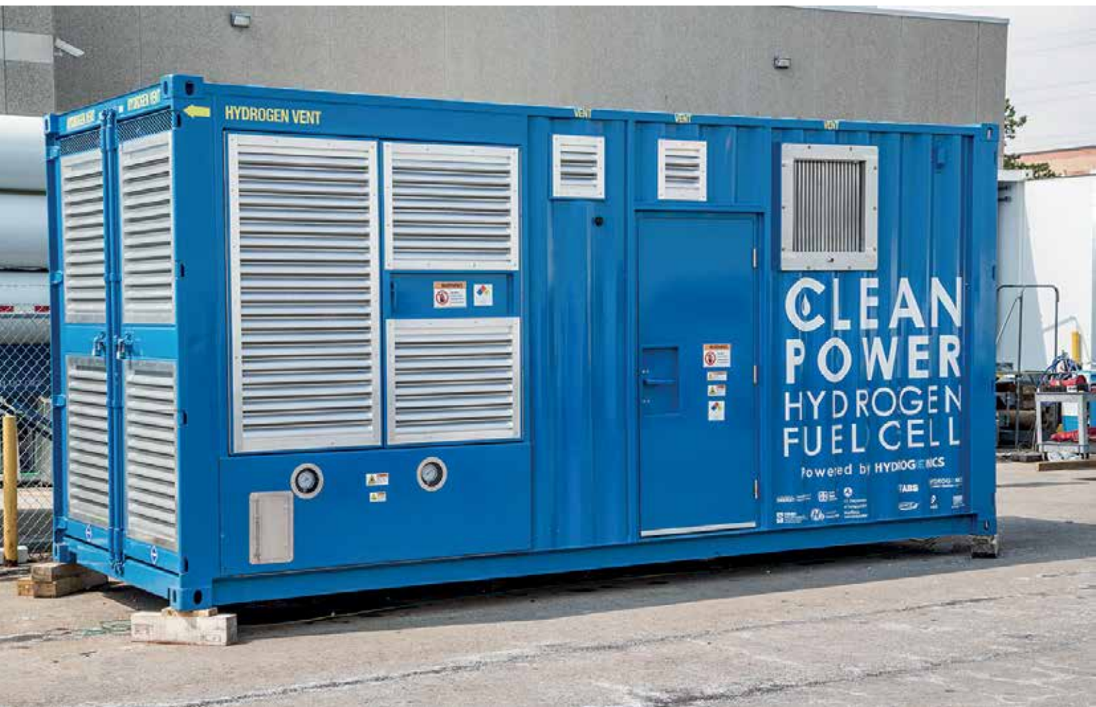
Figure 9: The Maritime Hydrogen Fuel Cell project in Honolulu, Hawaii. This hydrogen fuel cell consists of four 30 kilowatt fuel cells that are capable of providing bulk power.
