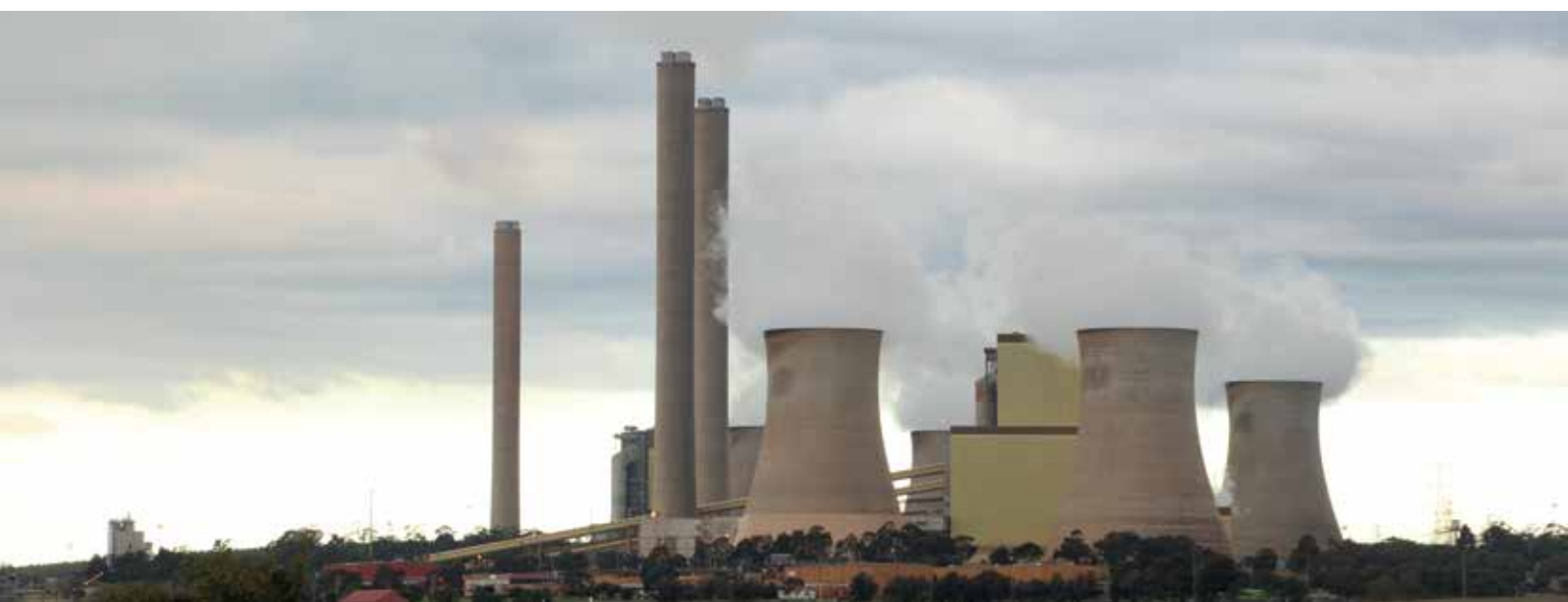
Figure 9: Australia's ageing and inefficient coal plants pose a threat to reliability.
