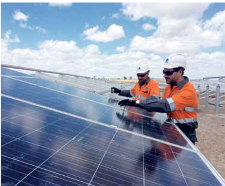
Figure 6: Workers at Lakeland Solar and Storage Project.
