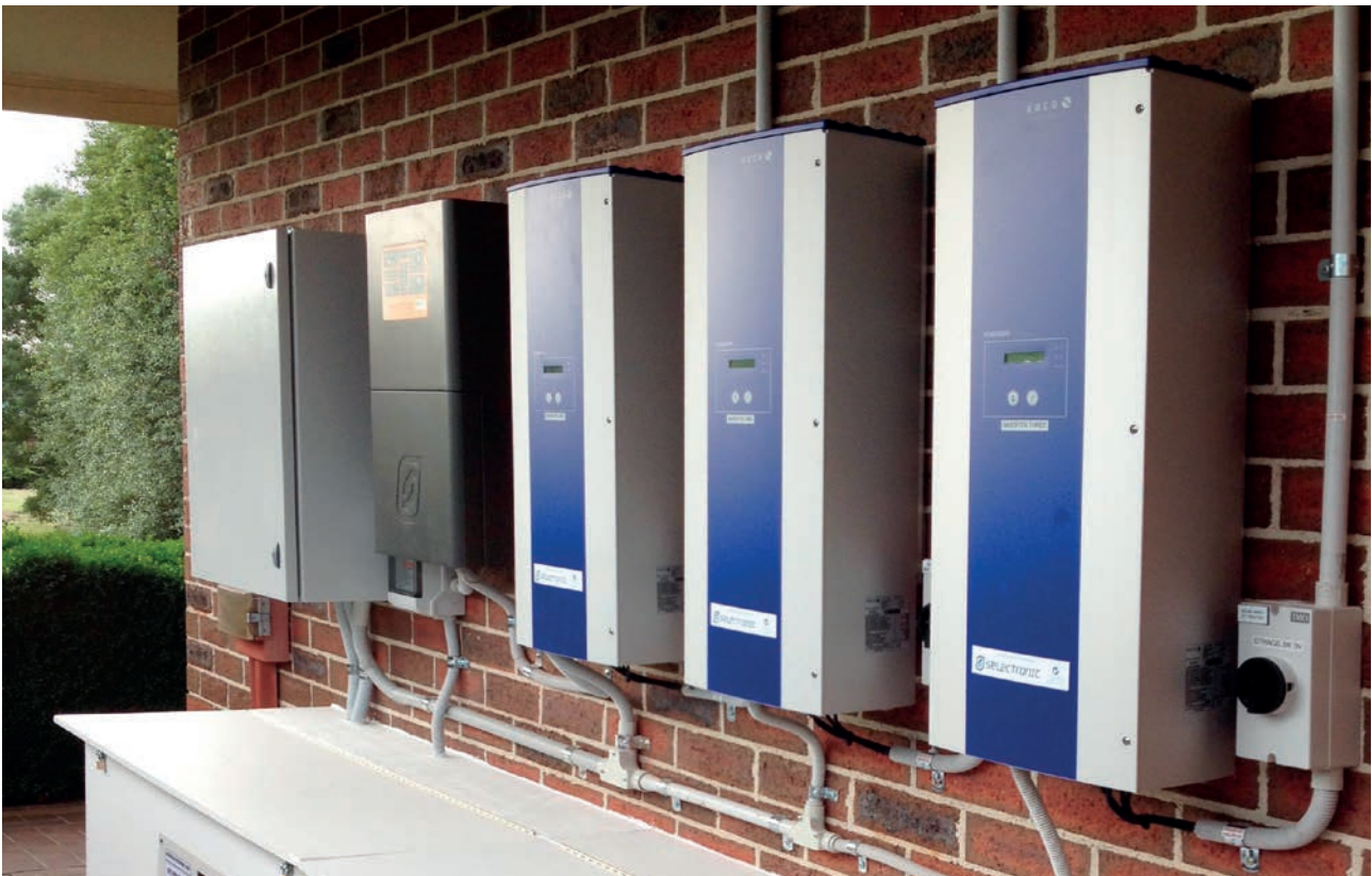
Figure 13: Household battery storage.
