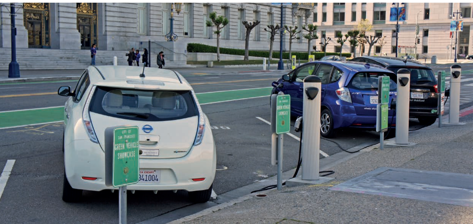
Figure 16: Electric cars at a public charging station at San Francisco City Hall.
