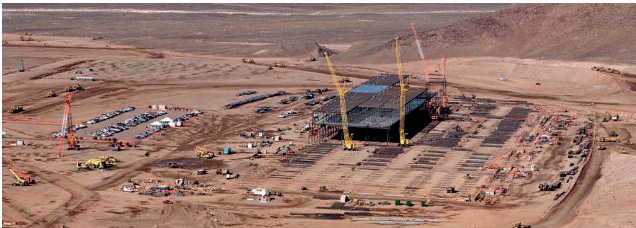
Figure 5: Tesla's "Gigafactory" under construction.
