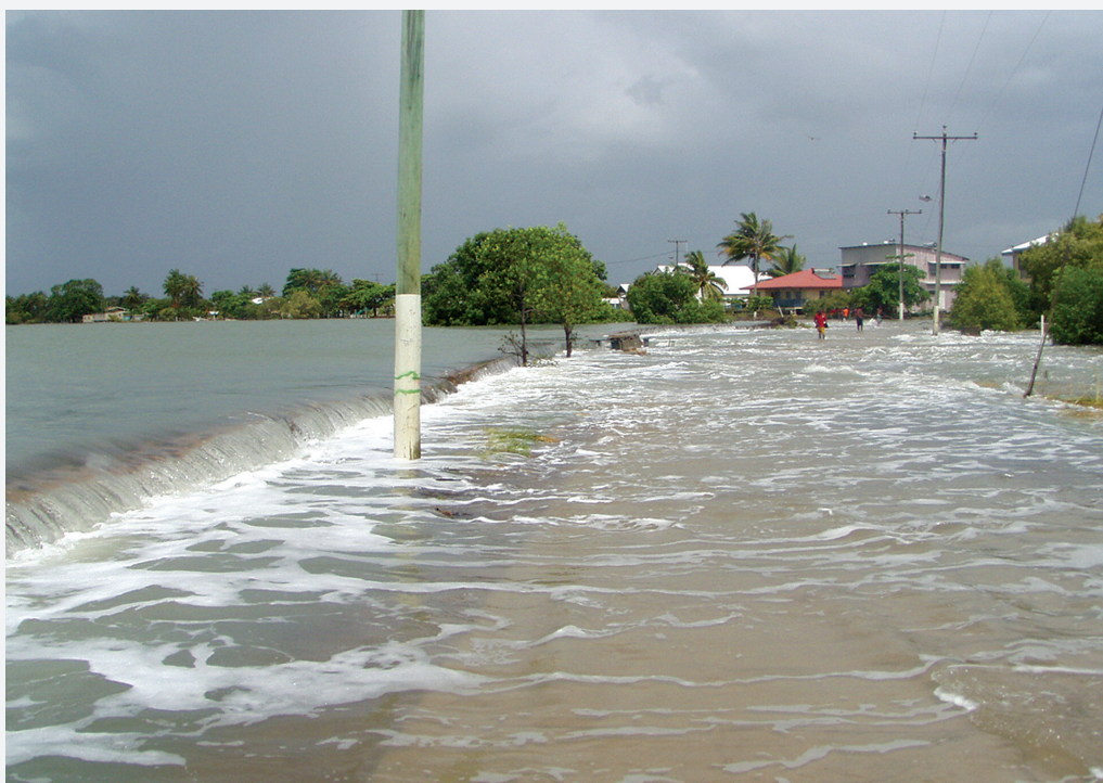
Figure 18: Seawater overflowing a protective wall, Saibai, Torres Strait Islands.
