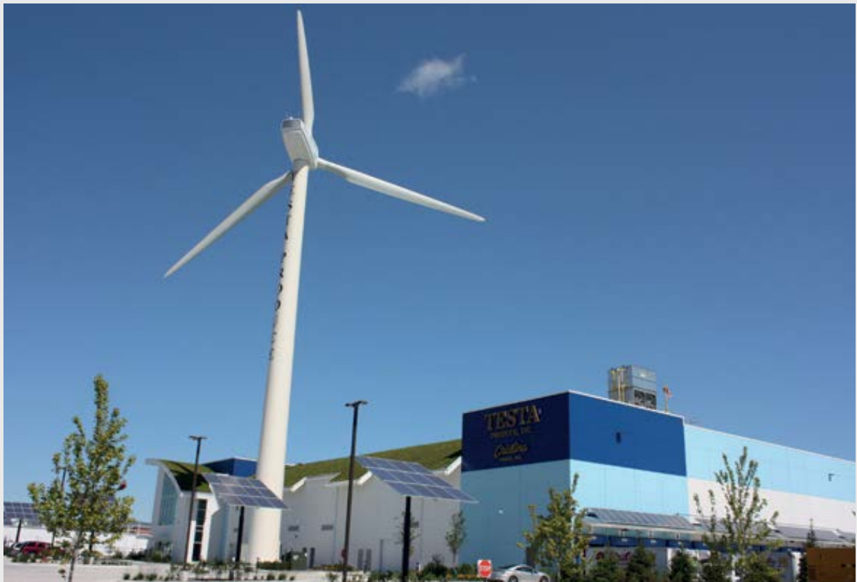
Figure 15: Refrigerated food distribution facility in Chicago with leading energy efficient design and onsite renewable energy.
