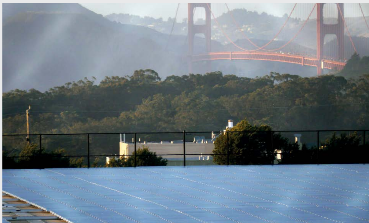
Figure 11: San Francisco, solar panels installed on a water reservoir.
