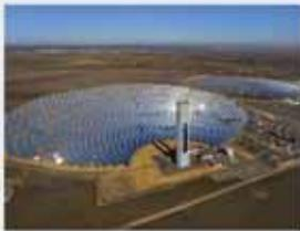
**Concentrated solar thermal:** Concentrated solar thermal is used to produce electricity on a large scale. Concentrated solar thermal uses mirrors to reflect sunlight into a small area to heat fluids or salts. These heated fluids then drive a steam turbine to create electricity. An advantage of concentrated solar thermal is that it can incorporate energy storage, meaning a power station can produce energy even when the sun is not shining.
