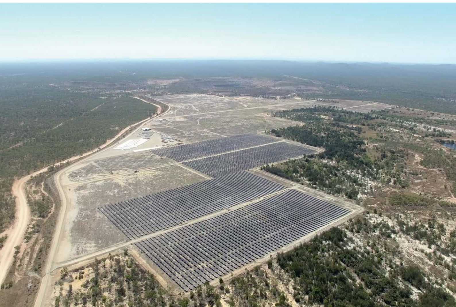
Figure 10: The Kidston Project in North Queensland combines solar power with pumped hydro energy storage utilising an abandoned Gold Mine.
