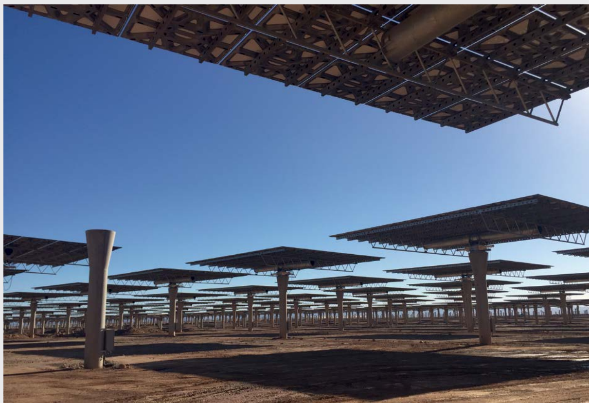
Figure 7: Morocco's Noor-Ouarzazate Solar complex.
