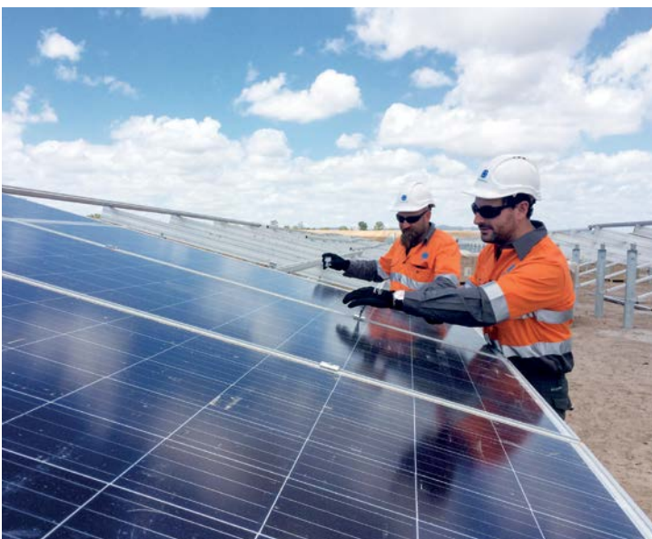
Figure 6: Workers at Lakeland Solar and Storage Project.
