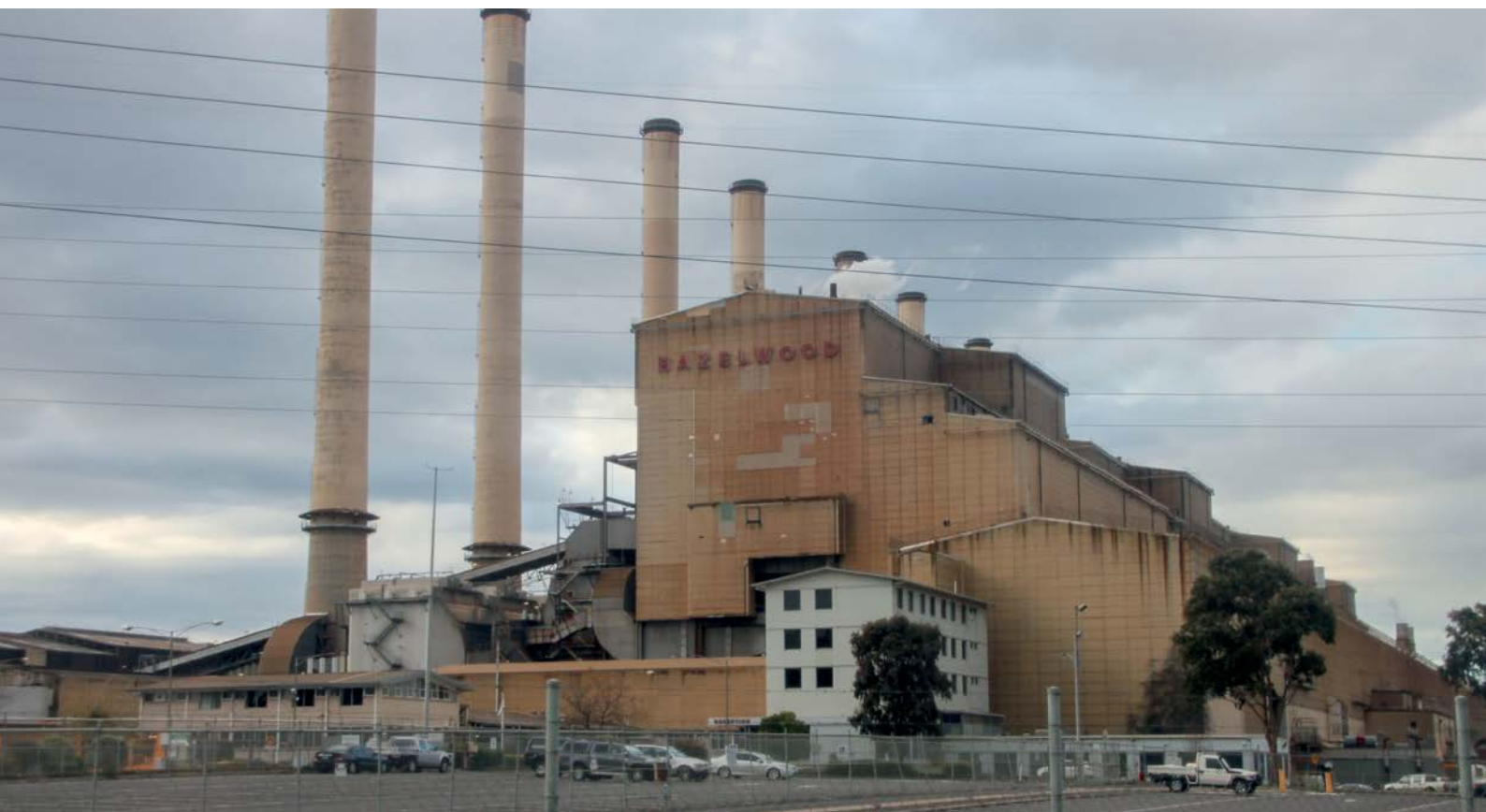
Figure 1: Hazelwood Power Station closed in March 2017.
