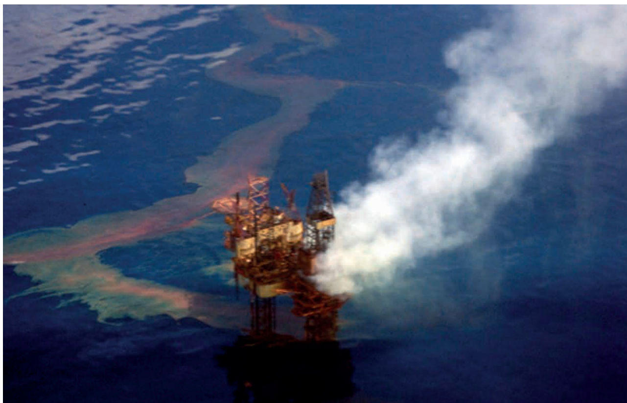
Figure 5: Montana gas and oil blowout shows the huge cloud of escaping vented gas and oil slick - the platform is not on fire at this stage.
