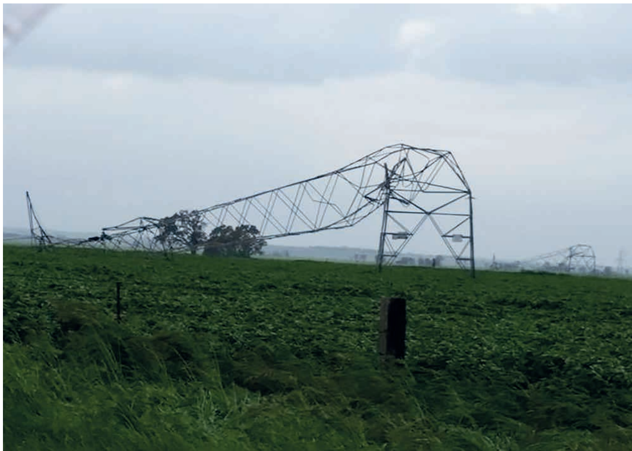
Figure 12: Severe storms in South Australia brought down transmission towers in 2016.
