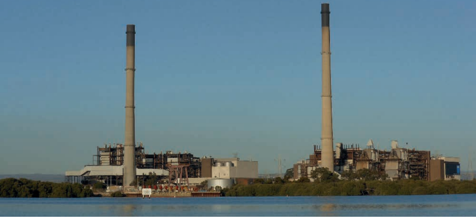
Figure 3: Torrens Island Power Plant, South Australia.
