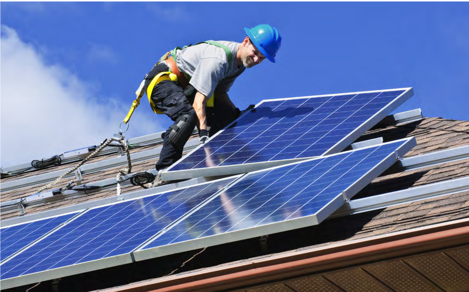
Figure 8: Worker installing household solar PV.
