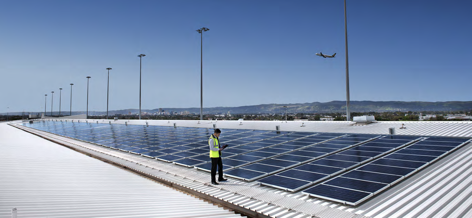
Figure 11: Adelaide Airport Solar PV panels.
