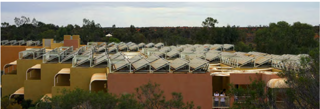
Figure 15: Solar panels on a hotel roof, Uluru, Northern Territory.
