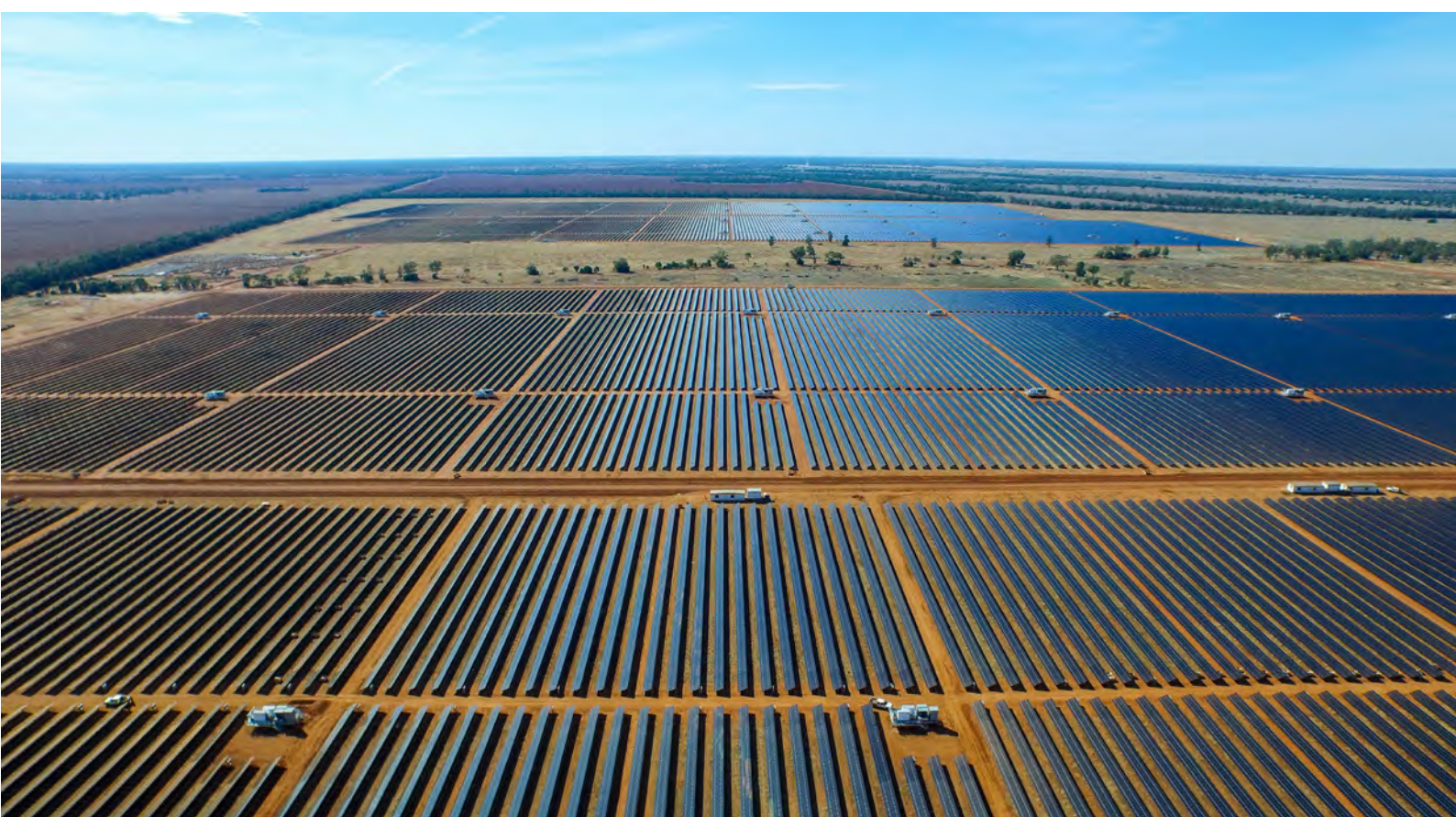
Figure 7: AGL's large-scale photovoltaic (PV) power plant in Nyngan, New South Wales.
