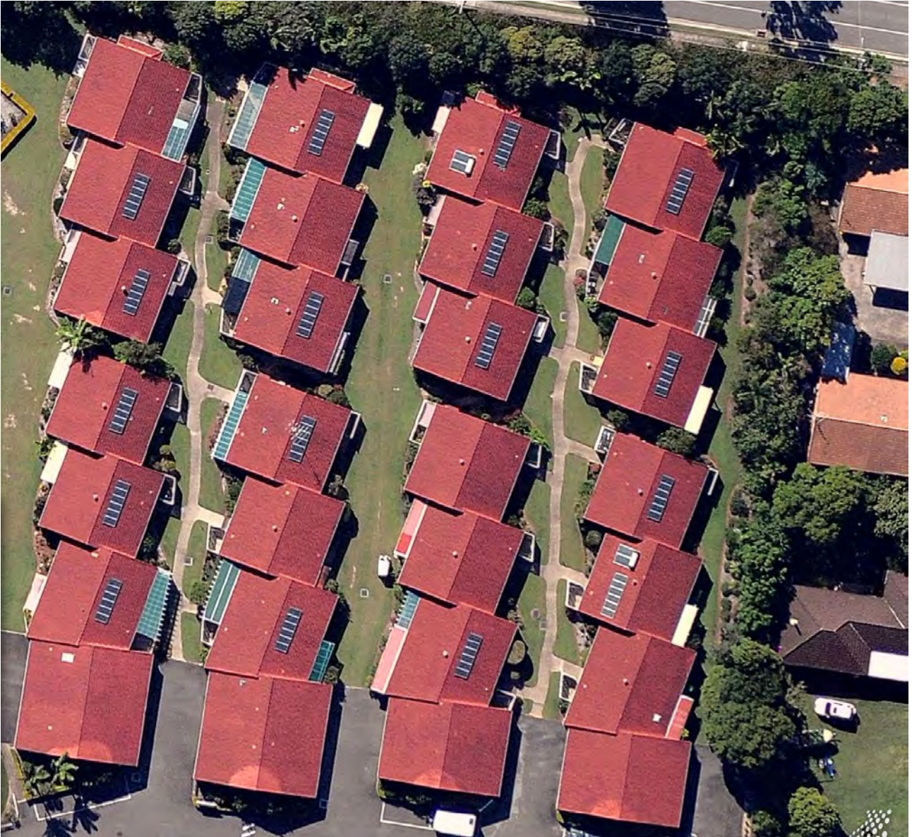
Figure 14: Rooftop solar panels in Beenleigh Queensland.
