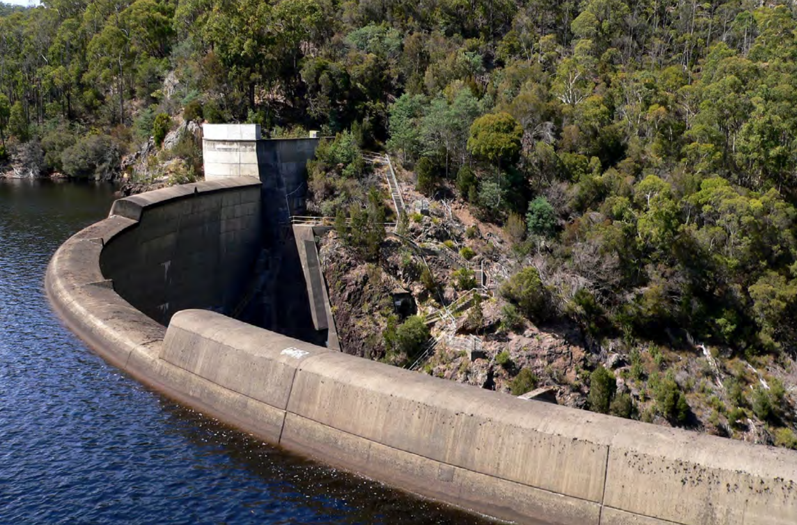
Figure 13: Hydro dam providing renewable energy in Tasmania.
