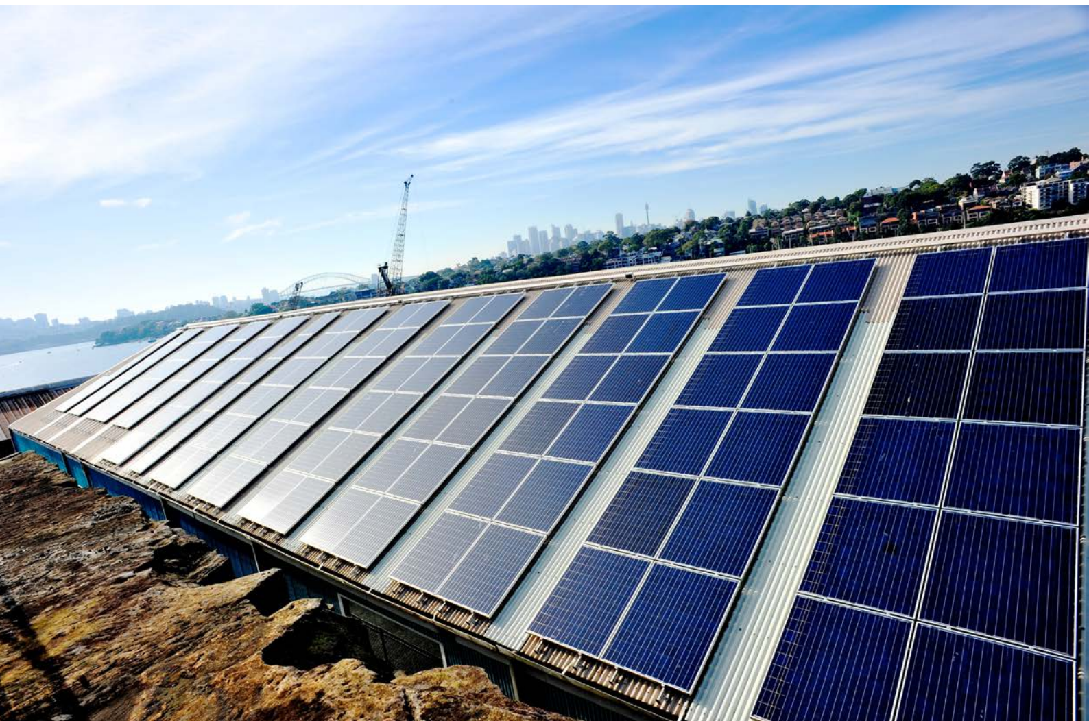
Figure 9: Solar PV panels in Sydney, generating renewable energy.
