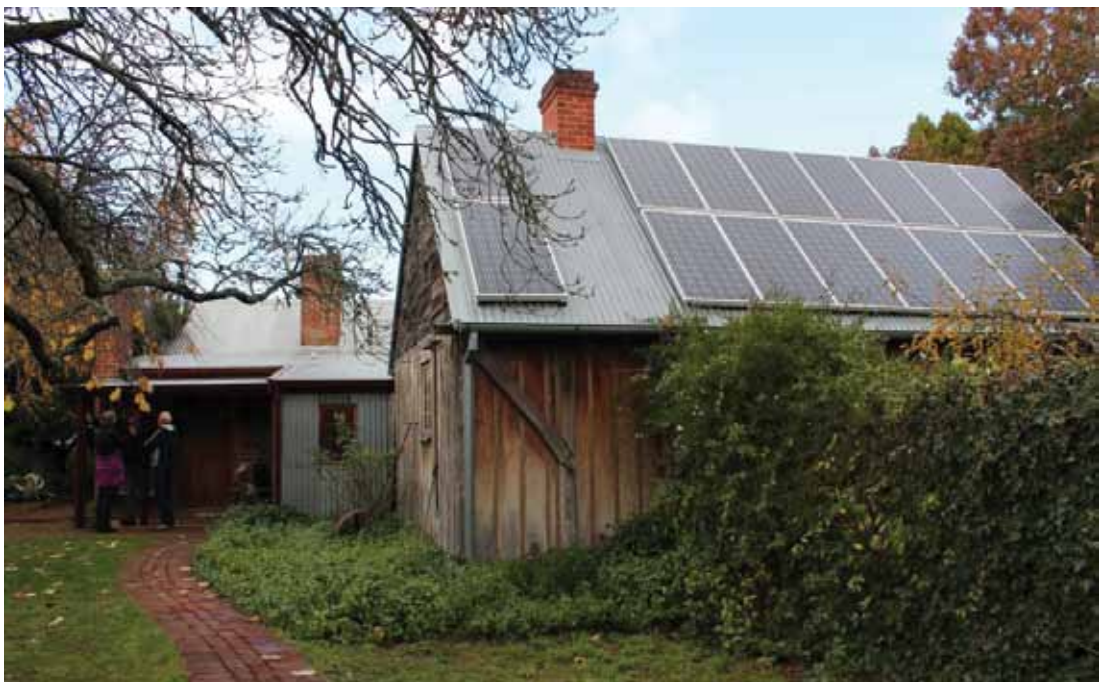
Figure 5: Solar PV on Hahndorf historic house, South Australia
