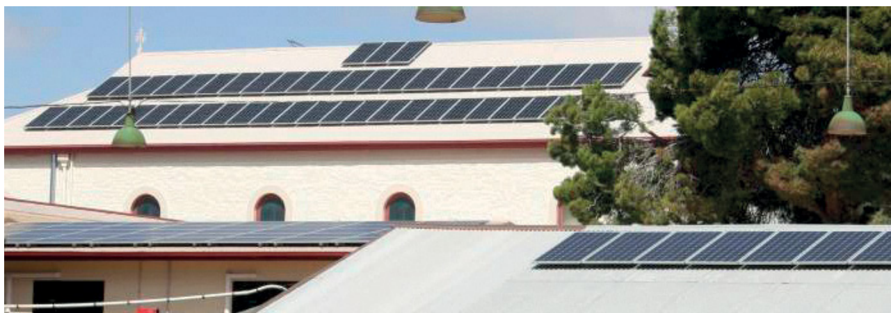
Figure 3: Solar rooftops in Melrose, South Australia.
