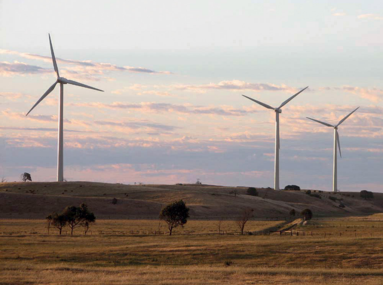
Figure 2: Wind farm near Millicent, South Australia.
