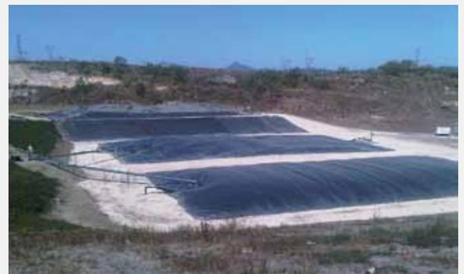
This photo shows three of the biocells at the Swanbank Renewable Energy Facility. Two contain organic waste and one contains leachates (liquid waste); the gas produced from the decay of this matter is collected by the pipes on the left of the photo.
