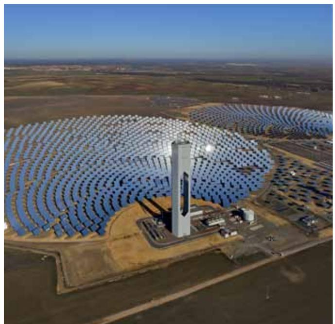
Concentrated solar thermal uses mirrors to reflect sunlight into a small area and heat fluids or salts.
