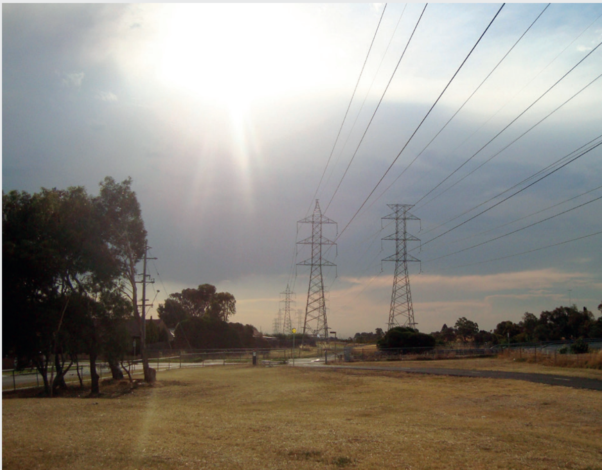
Figure 4: Extreme heat can cause severe impacts on infrastructure and essential services, including disruptions to electricity networks.
