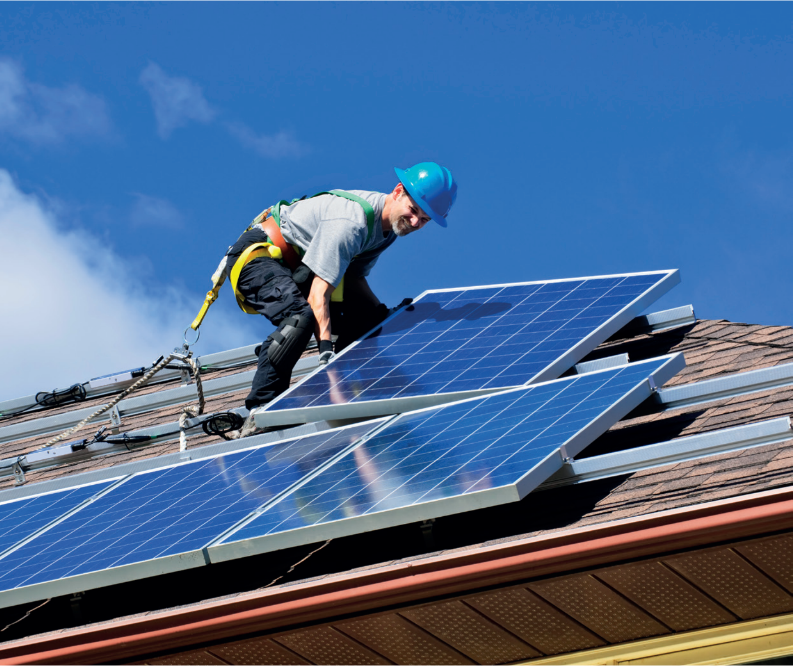
Figure 12: Installing rooftop solar.
