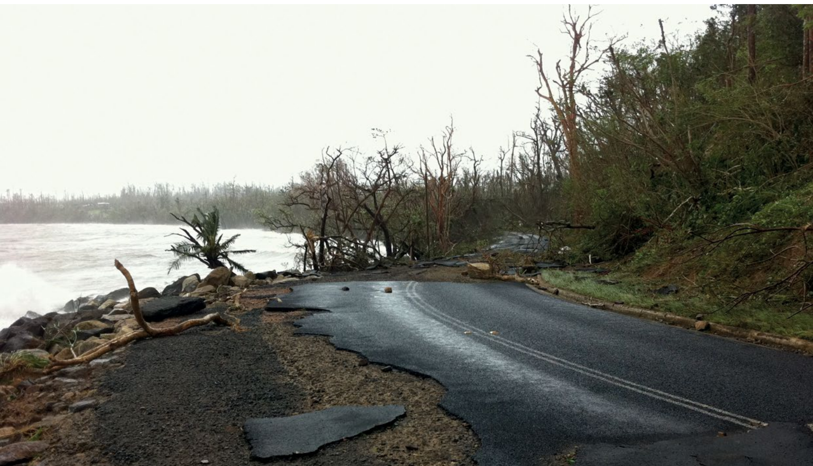
Figure 12: An example of damage to a road from coastal flooding at Mission Beach, in Queensland.
