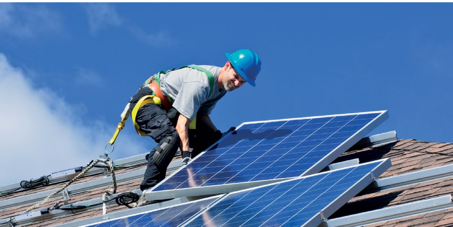
Figure 3: Worker installing solar panels on rooftop. Australia is a world leader; more than 30% of dwellings in Queensland and South Australia have rooftop solar.
