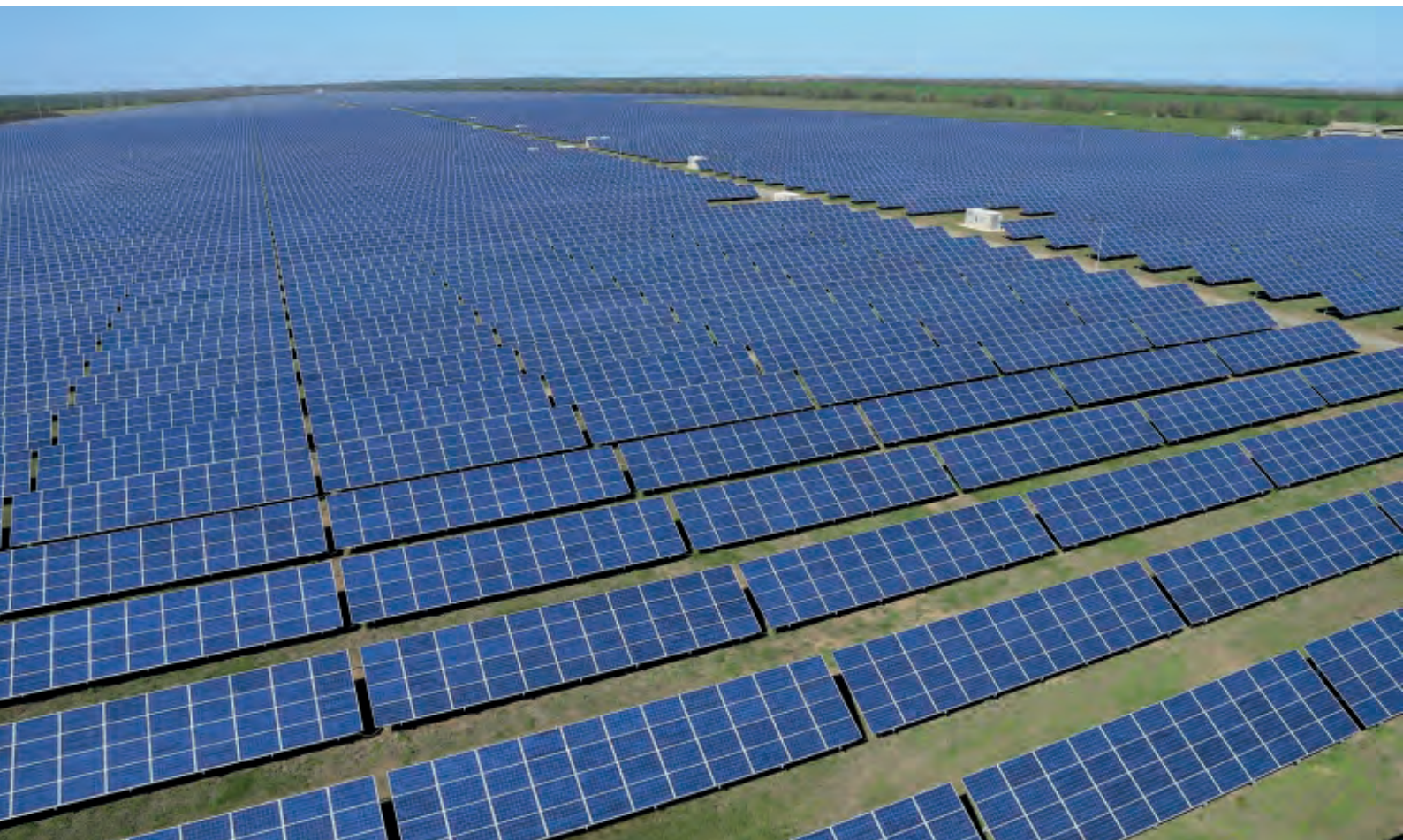
Figure 6: A large-scale solar farm (43MW) in southeastern Europe. More solar PV was added globally in 2016 than in any other year.
