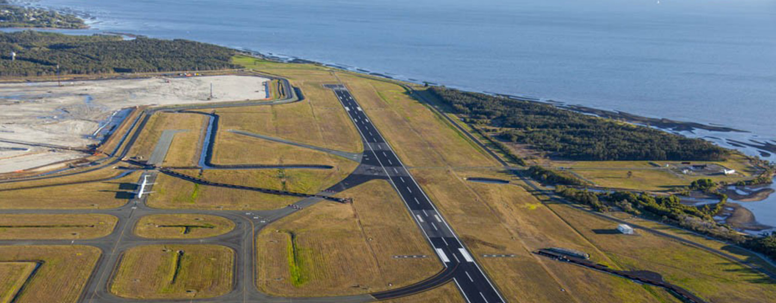
Figure 3: A cross-runway at Brisbane Airport, located on a low-lying site near Moreton Bay, with a new runway under construction (top left of photo). The design of Brisbane Airport's new runway, located on a low-lying coastal fringe, was informed by the latest sea-level science from CSIRO.
