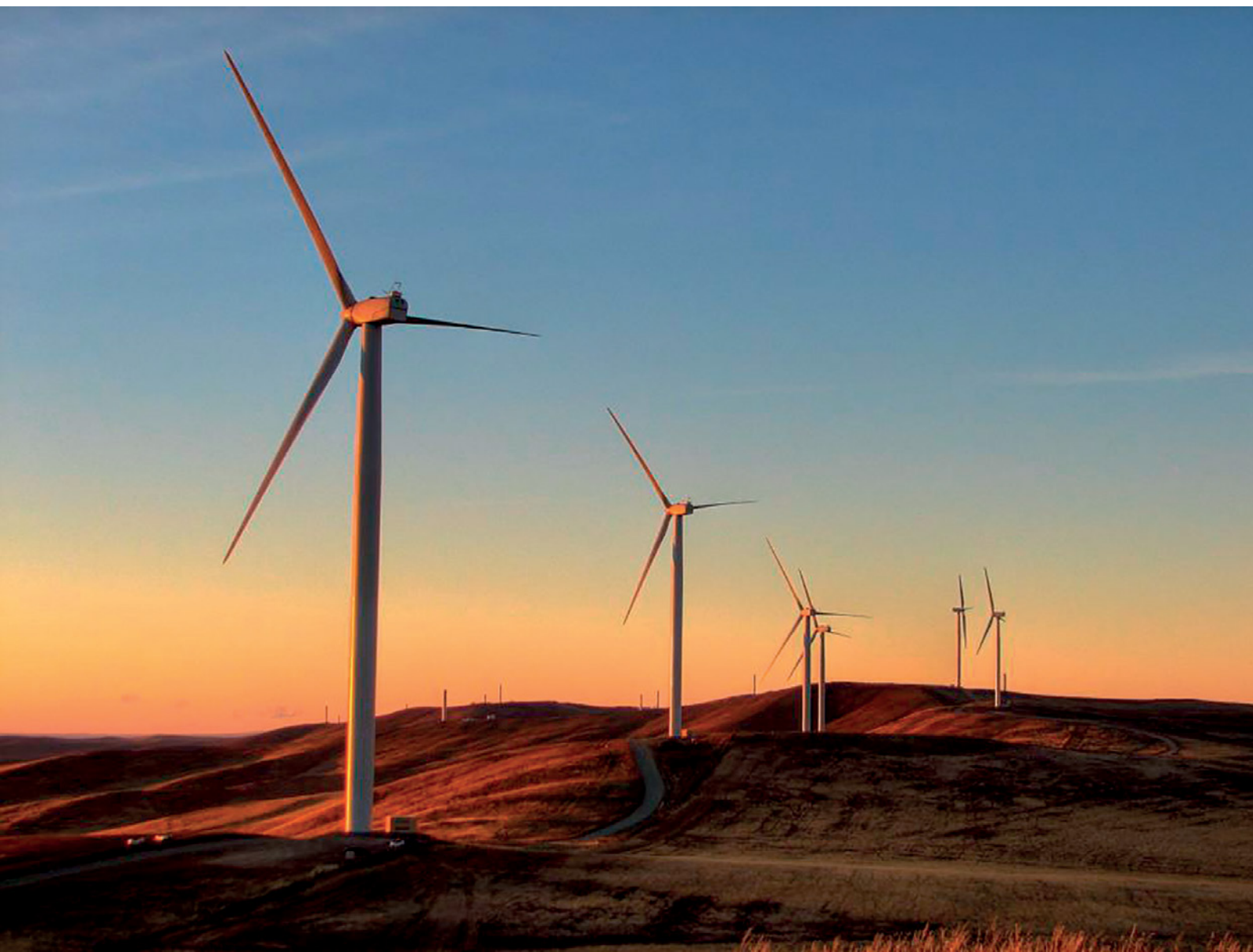
Figure 14: Wind turbines at Brown Hill Range, South Australia.
