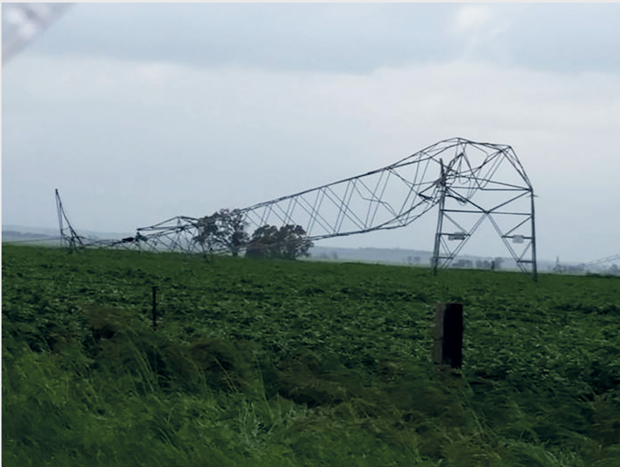
Figure 6: Catastrophic failure of transmission towers in the wake of the South Australian storm.
