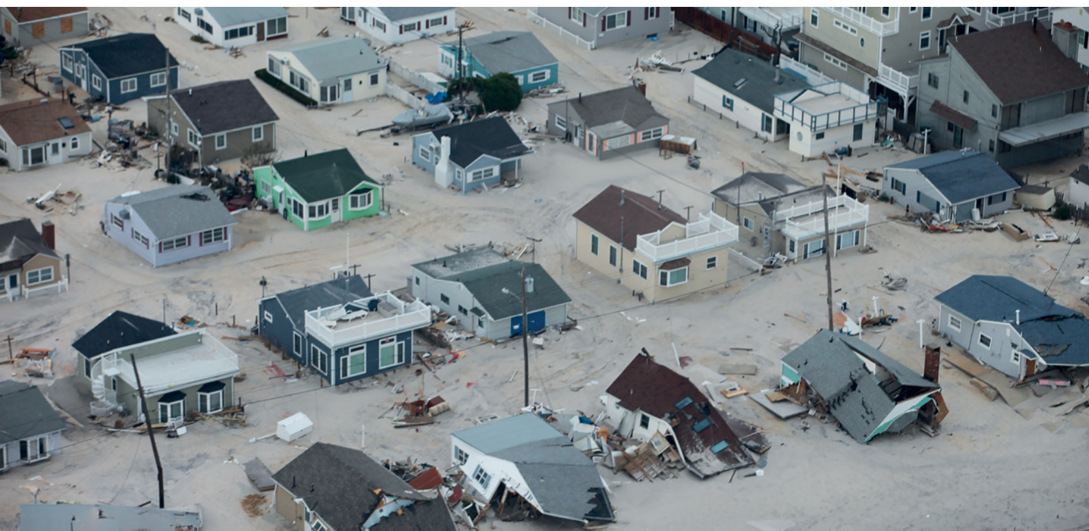
Figure 13: Aftermath of extensive flooding and coastal inundation along the New Jersey shore in November 2012 resulting from a storm surge driven by Hurricane Sandy.
