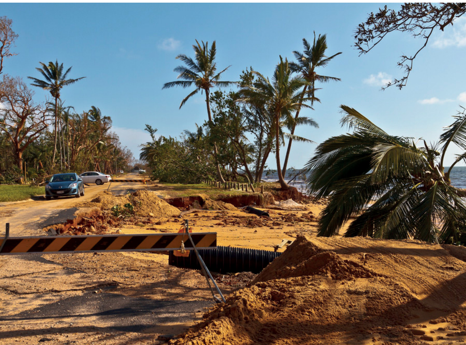
Figure 5: Some of the impacts of Cyclone Yasi which struck the north Queensland coast in 2011 included felled trees, beach erosion and damaged roads.
