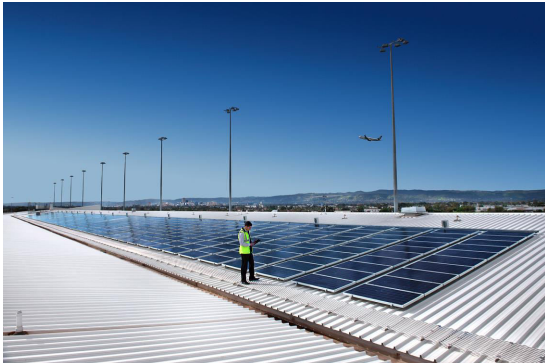
Figure 5 - Adelaide Airport Solar Panels. South Australia is on track to generate over 50% renewable energy by 2030.
