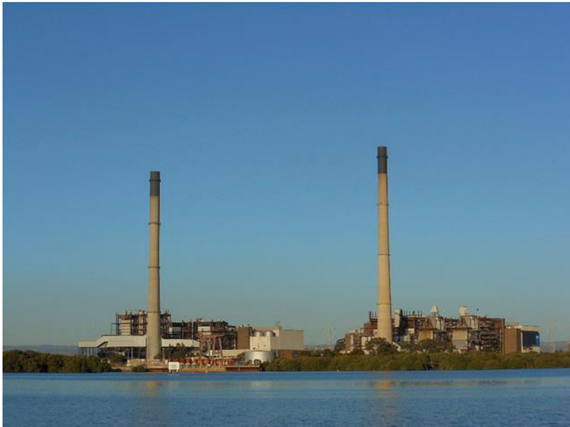
Figure 1 - Adelaide's Torrens Island Gas Power Station.
