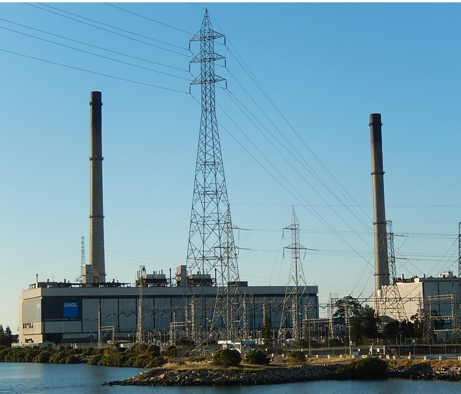
Figure 4: Torrens Island Power Station.
