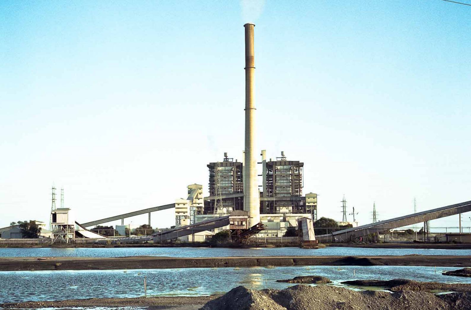
Figure 2: Northern coal-fired power station (now closed).
