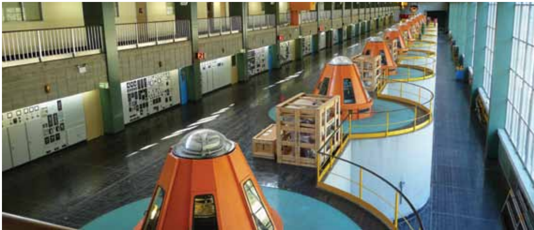
Figure 7: Snowy Hydro Scheme, New South Wales
