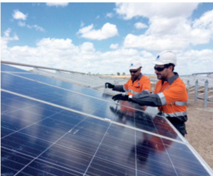
Figure 6: Workers at Lakeland Solar and Storage Project.
