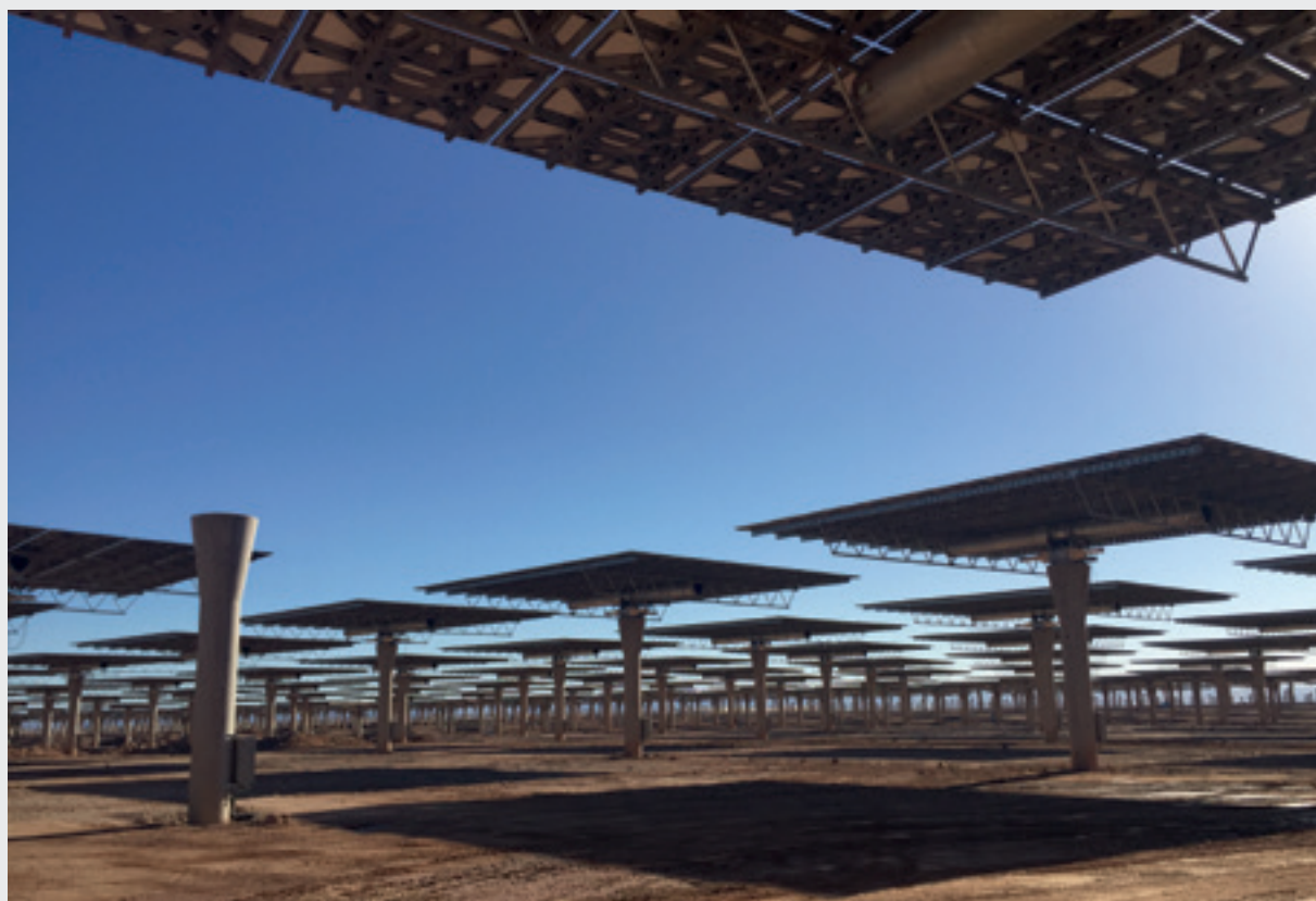
Figure 7: Morocco's Noor-Ouarzazate Solar complex.
