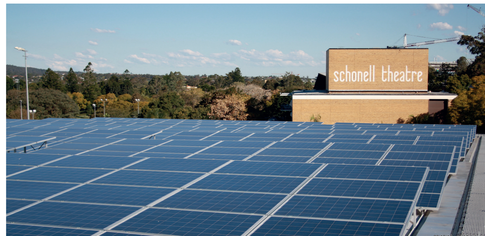
Figure 1: Rooftop solar at University of Queensland.
