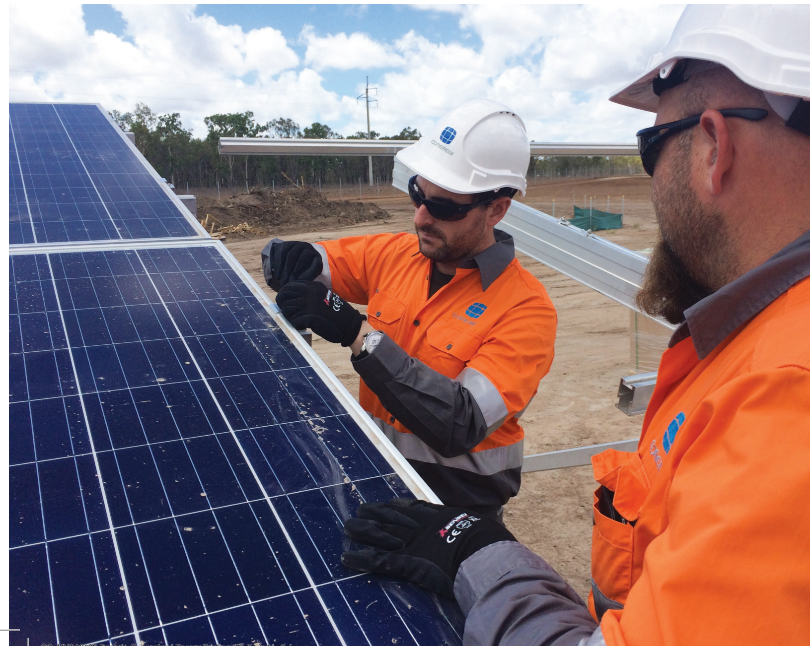
Figure 2: Lakeland Solar and Storage project under construction.
