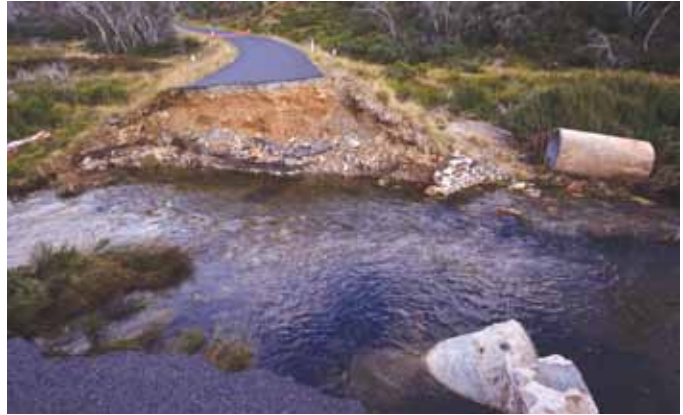
Figure 9. Floods can cause major damage to important infrastructure, such as roads and bridges.
