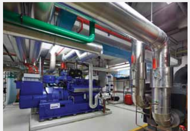
Figure 28. A trigeneration plant operating in an Investa-managed Sydney building.
