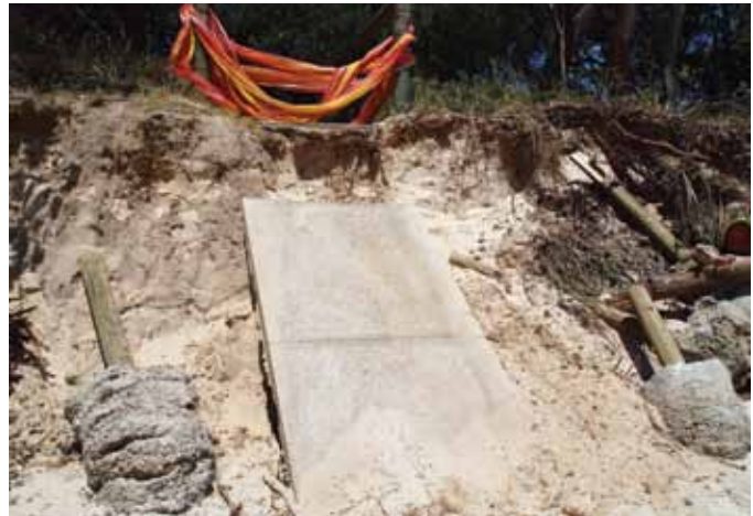
Figure 14. Erosion of coastal walkway at Scotts Head, NSW.
